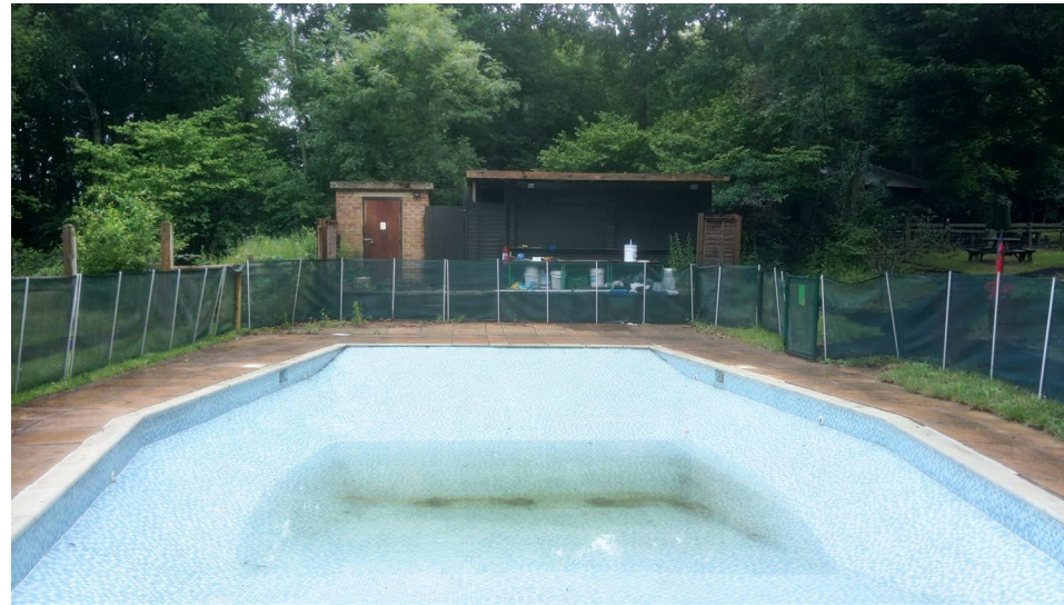
Figure 1. The pool and existing old buildings (looking north)
