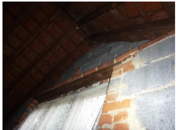
Photograph 12. Window in front gable.
