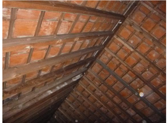
Photograph 10. Unlined roof.
