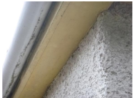
Photograph 6. Intact and tight timber soffits.
