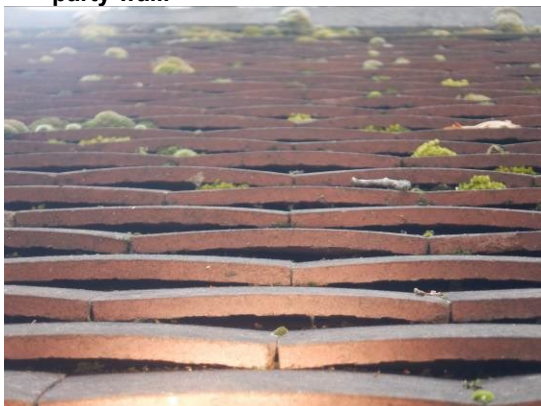
29. Gaps beneath curved tiles inspected (Sept 23)
