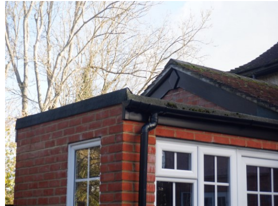
16. Bitumen felt tight to the brick wall of the flat roof section, viewed from the northwest.
