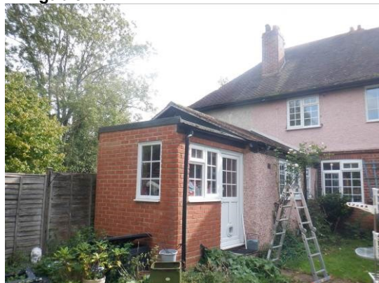
28. The single storey extension to be extended (Sept 23).
