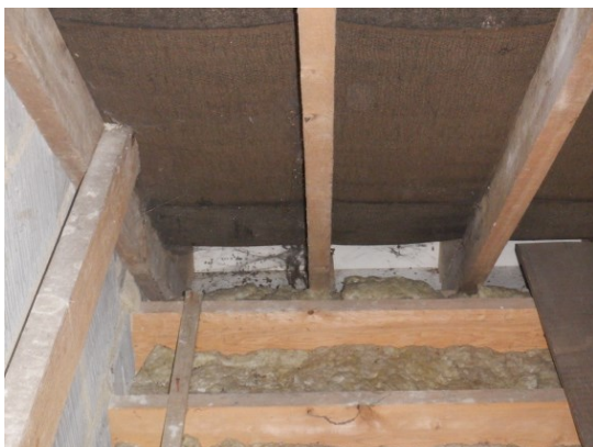
21. Open eaves within the southwest section of the roof void.
