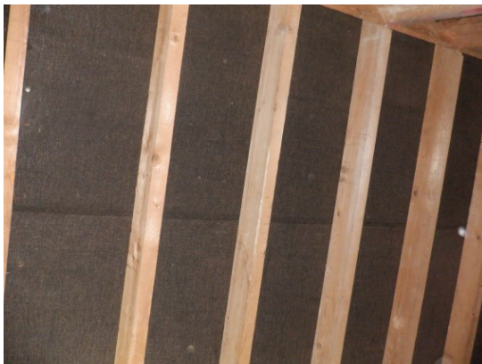
17. Type 1F bitumen felt mostly intact throughout the roof void.
