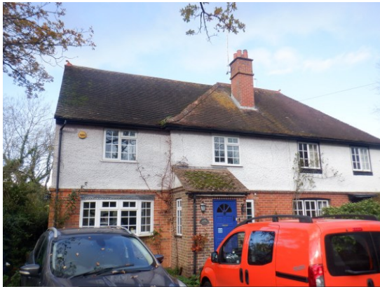
1. Front of the property, viewed from the southeast.
