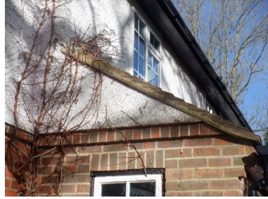
14. Verge mortar fully intact on front porch, viewed from the southwest.
