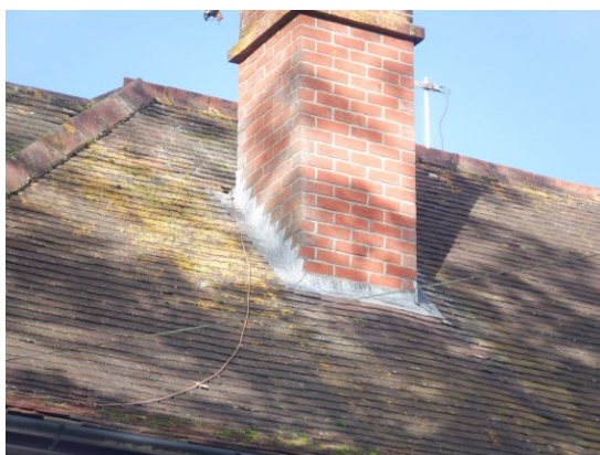
9. Tight lead flashing but gap between clay roof tiles and lead flashing to the rear of the chimney, viewed from the southeast.
