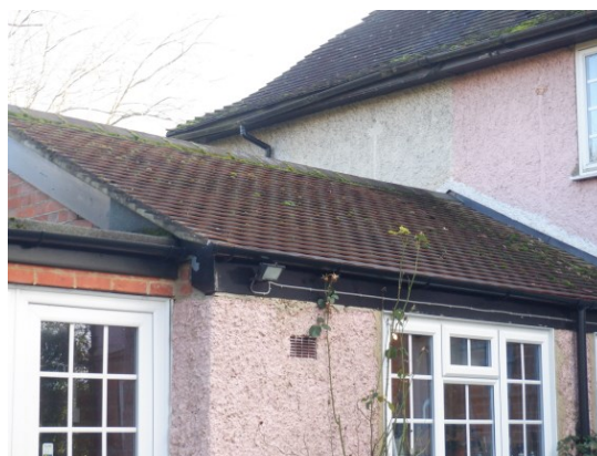
8. Verge mortar and ridge tiles fully intact on the existing rear extension, viewed from the west.
