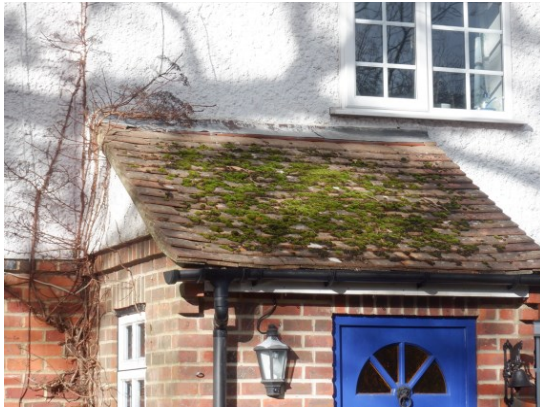
15. Occasionally lifted clay roof tiles under moss with lead flashing flush to the rendered wall, viewed from the southeast.
