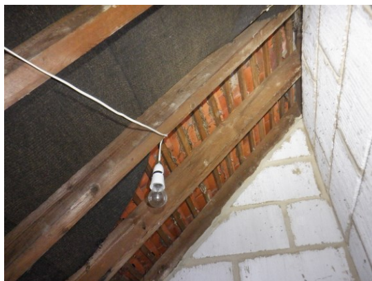
22. End rafter sealed to the northeast party wall.
