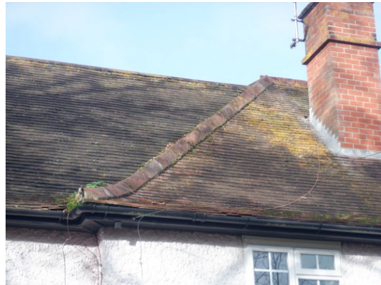
6. Mortar along the hip & ridge tiles fully intact, viewed from the southeast.
