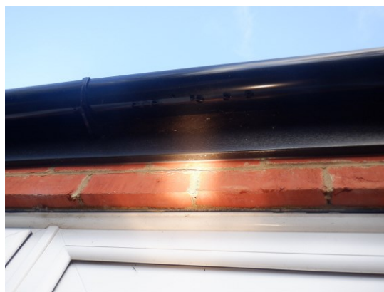
12. Timber fascia flush to the wall of the existing rear extension, viewed from the west.
