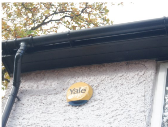
11. Timber soffit flush to the rendered wall of the main house, viewed from the southeast.
