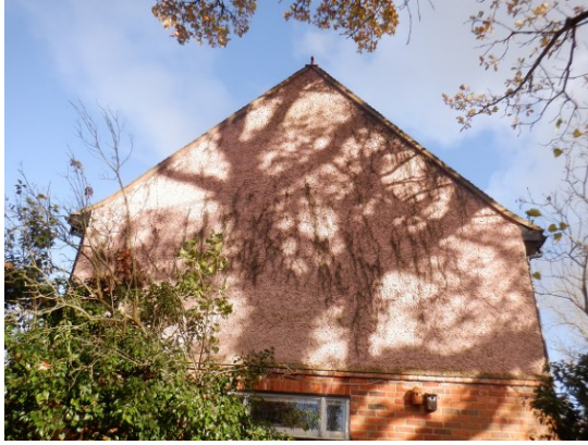
13. Two bird boxes on the southwest side elevation.
