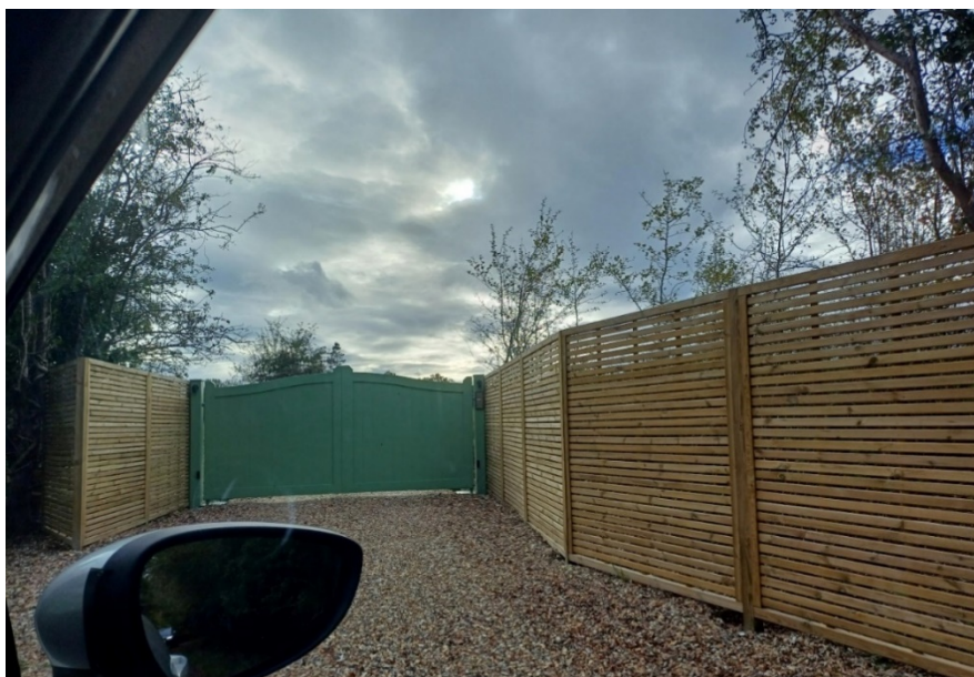
Photo taken 21.10.2025– Shows the new access gates and fence panels and the beginning of the gravelled access road
