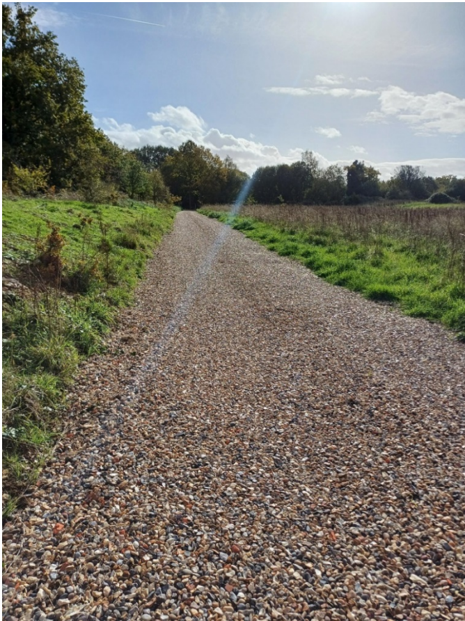
Photo taken 28.10.2025- shows gravelled access road
