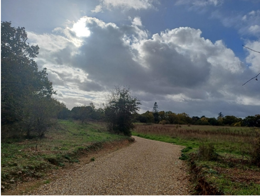
Photo taken 28/10/2025- Shows the gravelled access road
