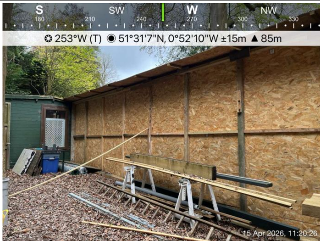
Photo 3: Southeast elevation of B1
