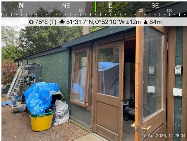
Photo 1: Northwest elevation of B1
