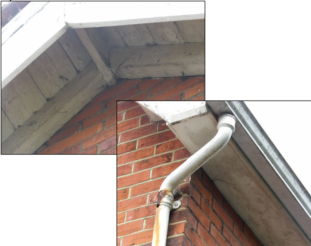
Figure 9. Example sealed eaves/soffits/fascias on property. Milverton, 38 New Road, Twyford. 10.06.25
