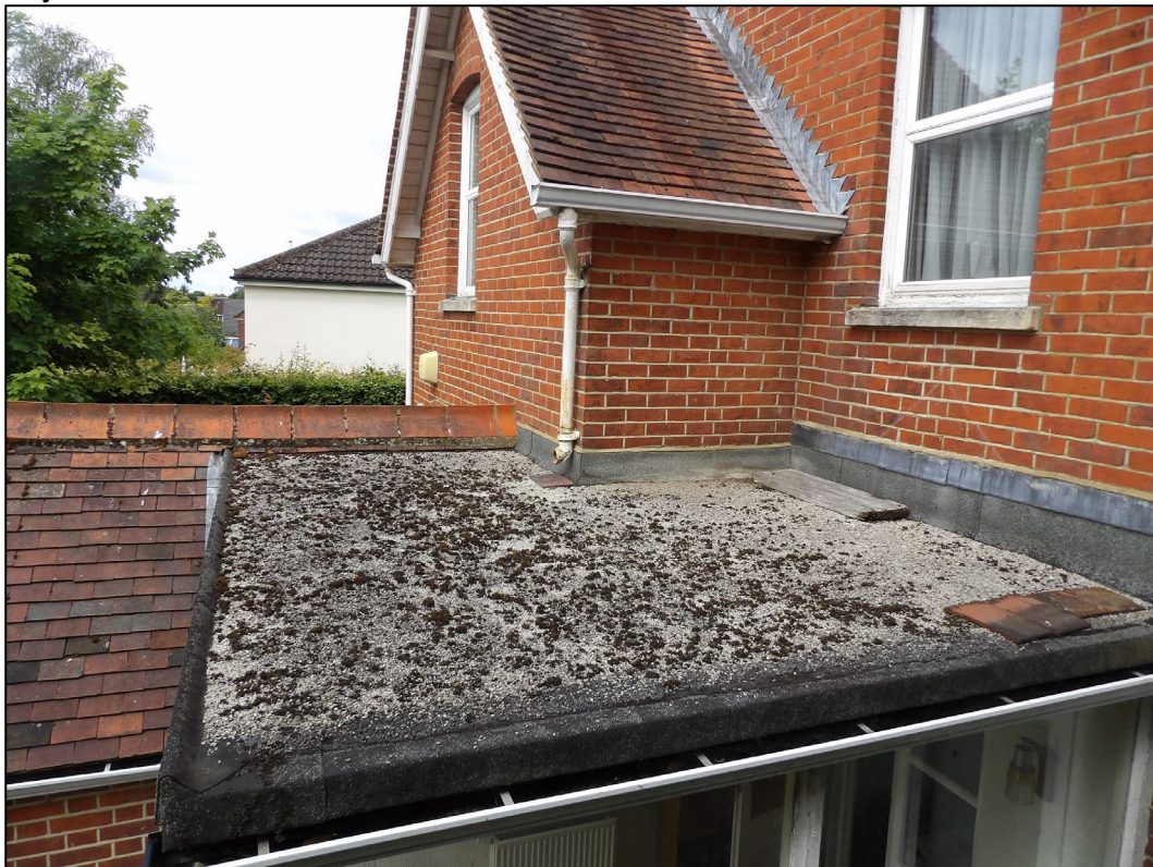
Figure 11. Well-sealed bitumen felt on rear extension. Milverton, 38 New Road, Twyford. 10.06.25
