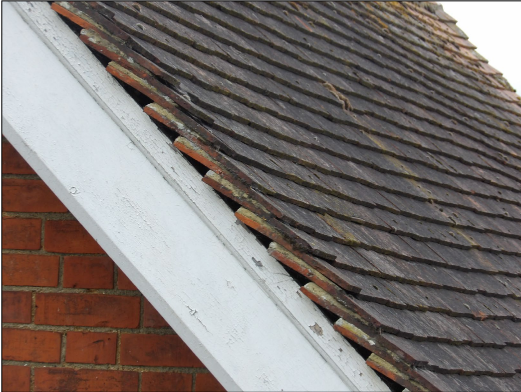
Figure 8. Example missing mortar from front verge. Milverton, 38 New Road, Twyford. 10.06.25
