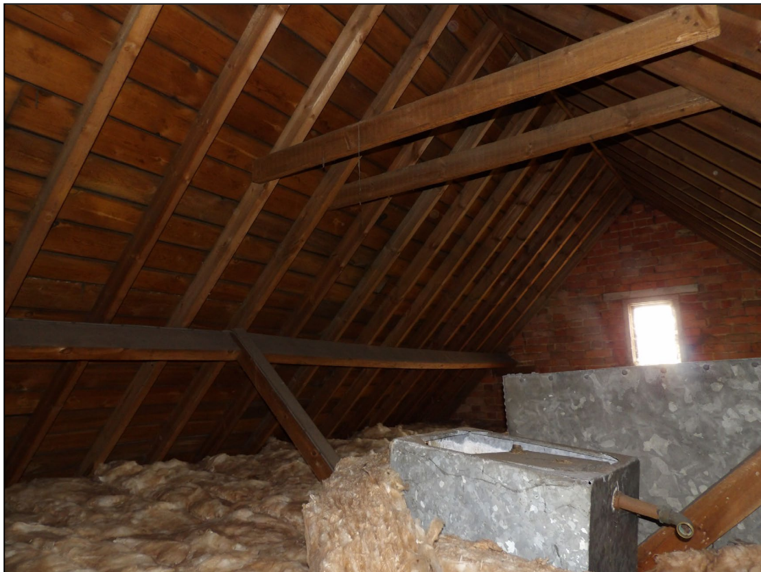
Figure 14. Example loft space and timber sarking. Milverton, 38 New Road, Twyford. 10.06.25
