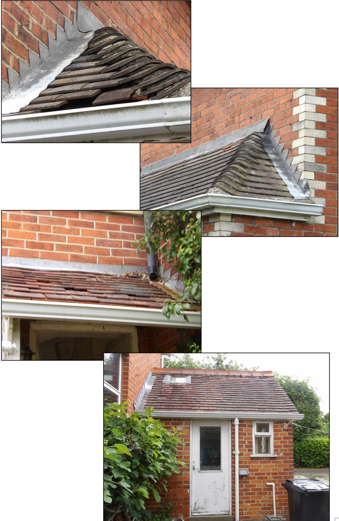
Figure 7. Example missing tiles and lifted lead flashing on bay window on eastern elevation. Missing tiles on the porch on western elevation and lifted tiles on rear, single storey pitched roof section. Milverton, 38 New Road, Twyford. 10.06.25
