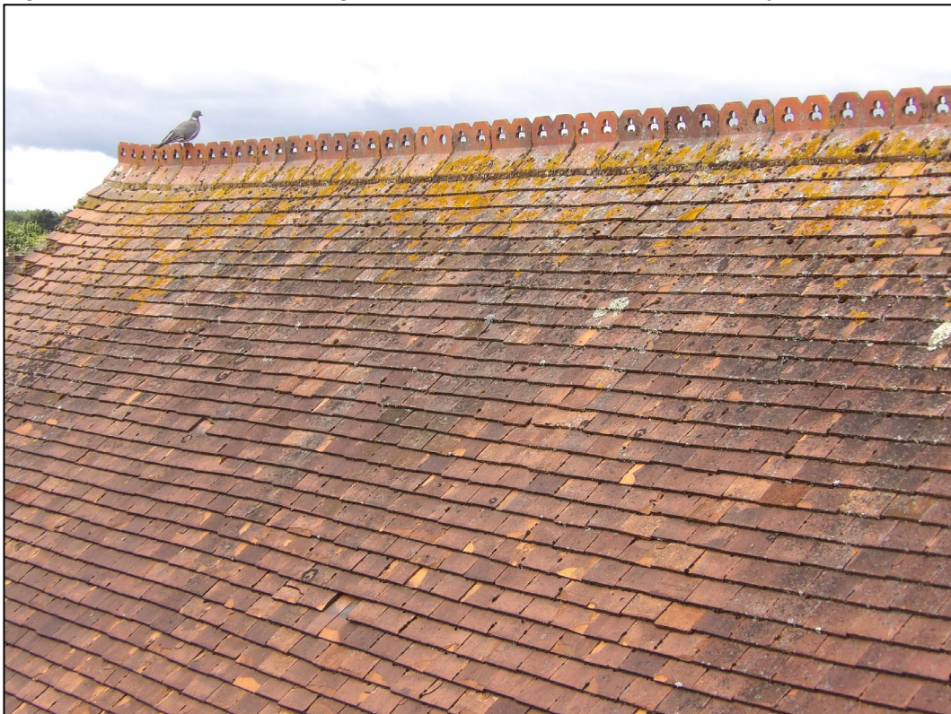
Figure 6. Example sealed ridge tiles. Milverton, 38 New Road, Twyford. 10.06.25
