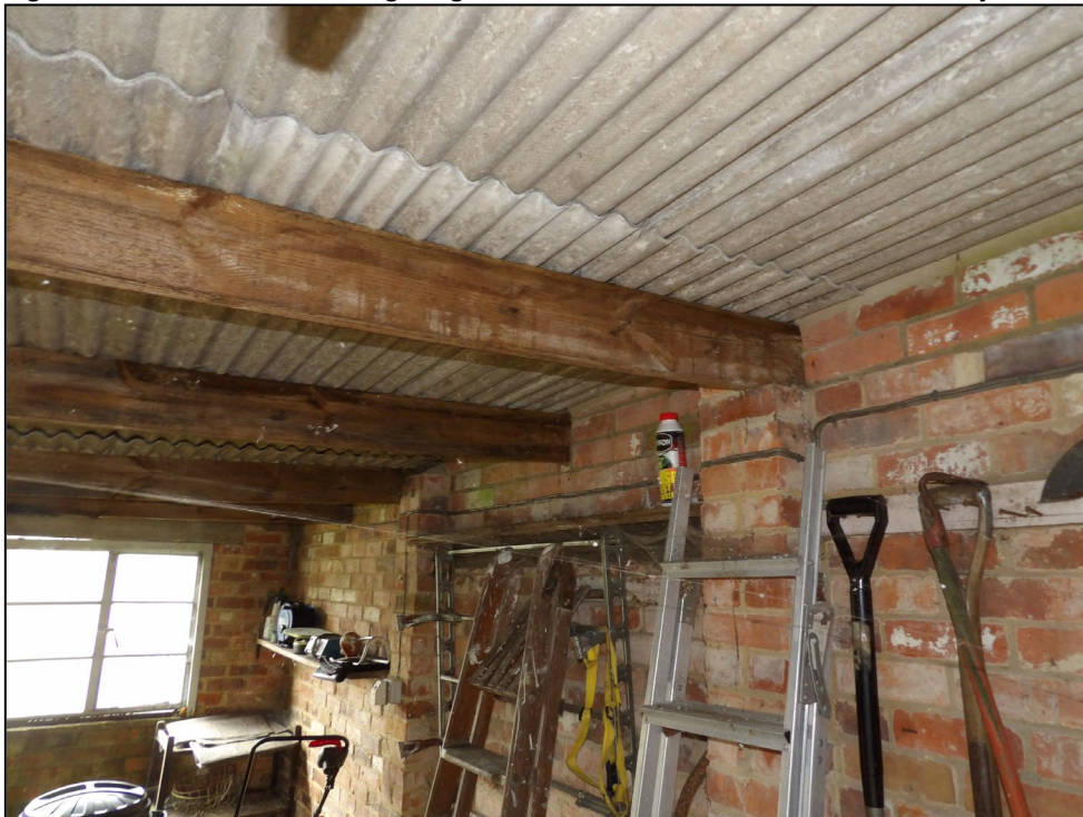
Figure 16. Internal view of garage roof. Milverton, 38 New Road, Twyford. 10.06.25
