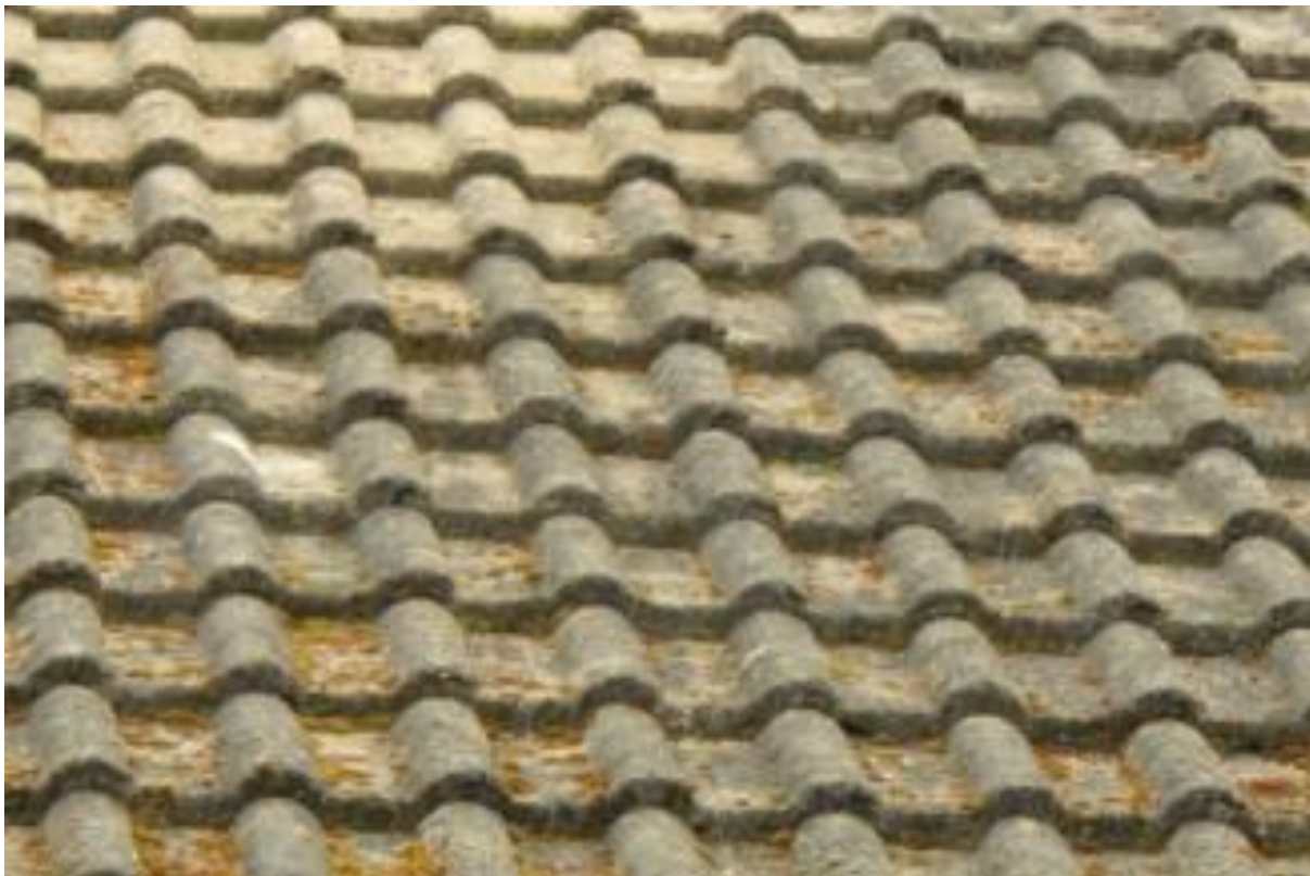
Image 2 – View of the front North facing roof coverings which have demonstrated a fair level of condition throughout
