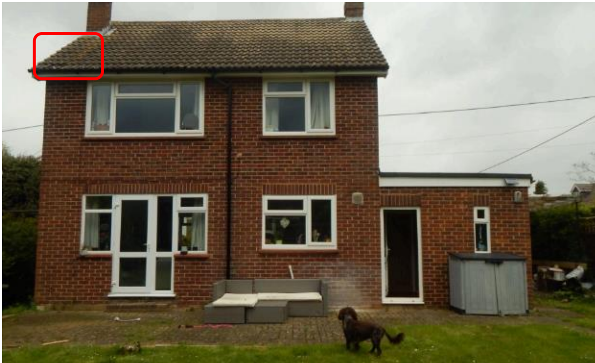
Image 3 – Rear South facing elevation of the property offering an area of raised tiles of adequate proportions to offer likely shelter/access opportunities for bats
