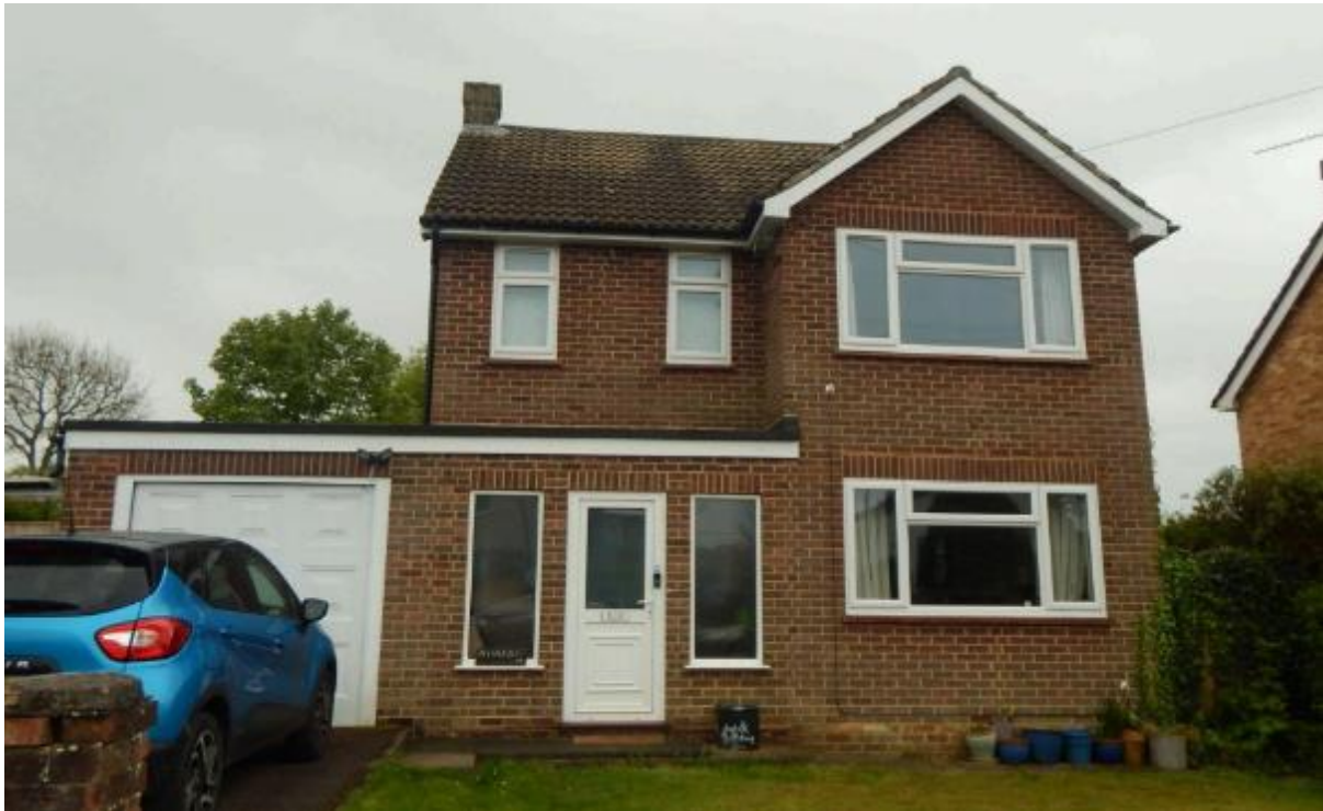
Image 1 – North facing elevation of the property.
