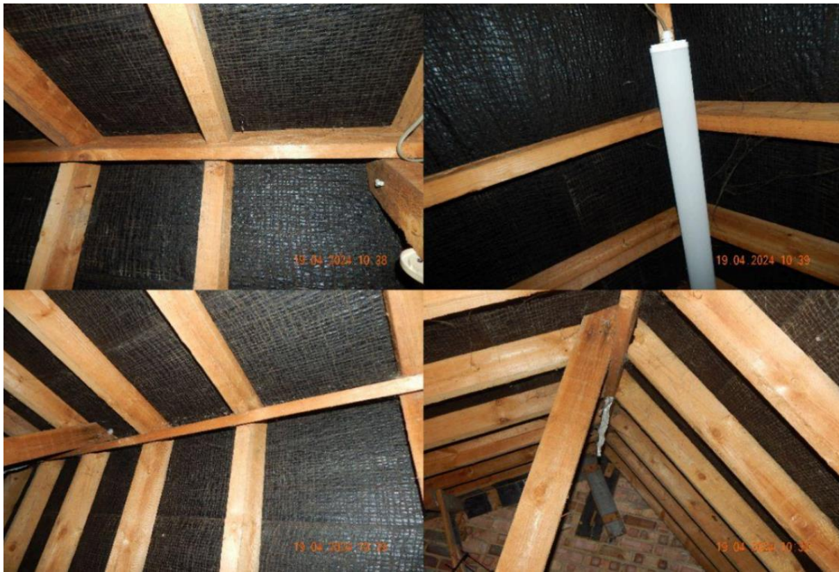
Image 9 – Internal view from within the main roof void spaces of the property
