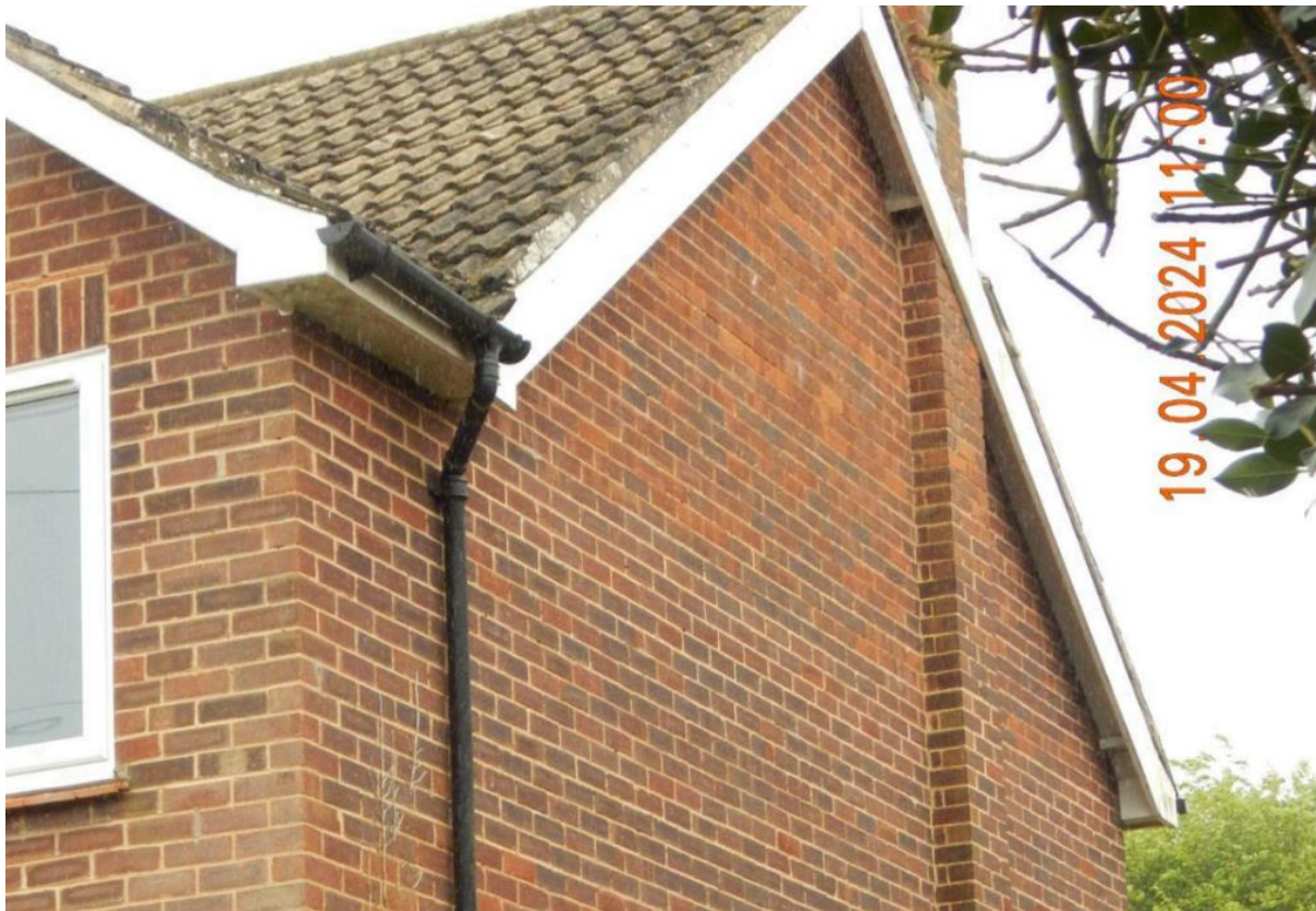
Image 7 – West facing elevation of the property
