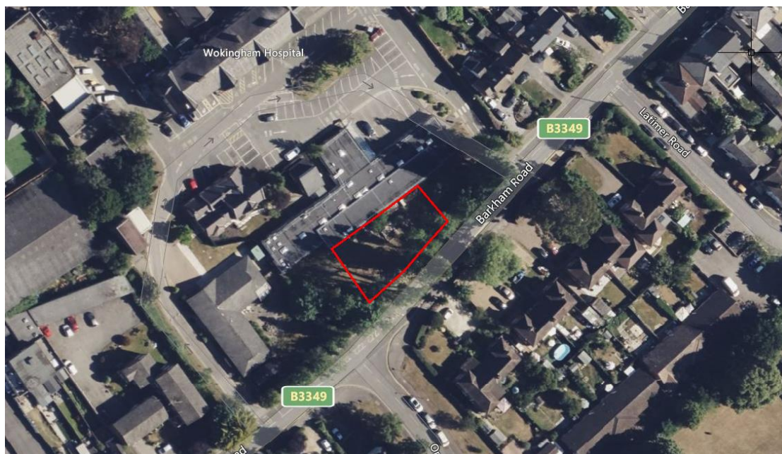
Figure 1: Site location shown on Google aerial image
