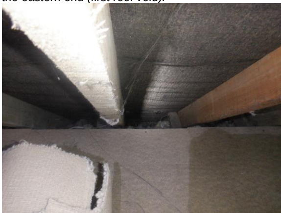
Photograph 15. Open eaves (first roof void).
