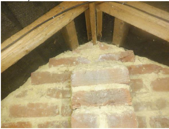
Photograph 19. Intact mortar on brickwork rear gable (Second roof void).
