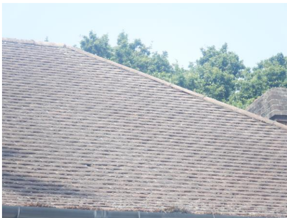
Photograph 4. Tight roof tiles and intact hip tiles and mortar on the house (rear elevation).
