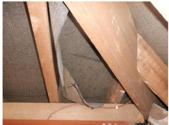
Photograph 14. Overlapping bitumen roofing felt at the western end (first roof void).
