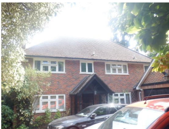
Photograph 1. Front of property viewed from the north.
