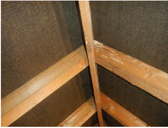
Photograph 17. Lightly cobwebbed ridge (Second roof void).
