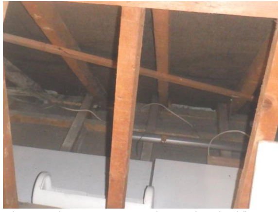
Photograph 18. Open eaves (Second roof void).
