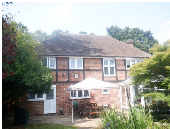
Photograph 2. Rear of property viewed from the south.
