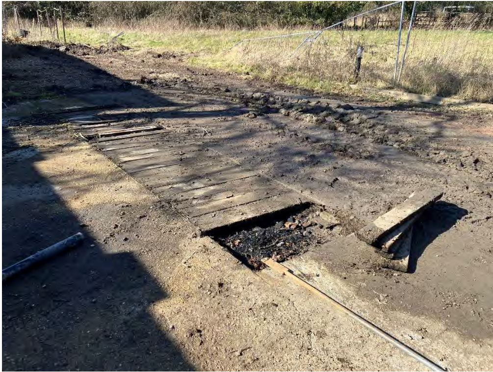
View of the covered and backfilled vehicle service pit (HA1)
