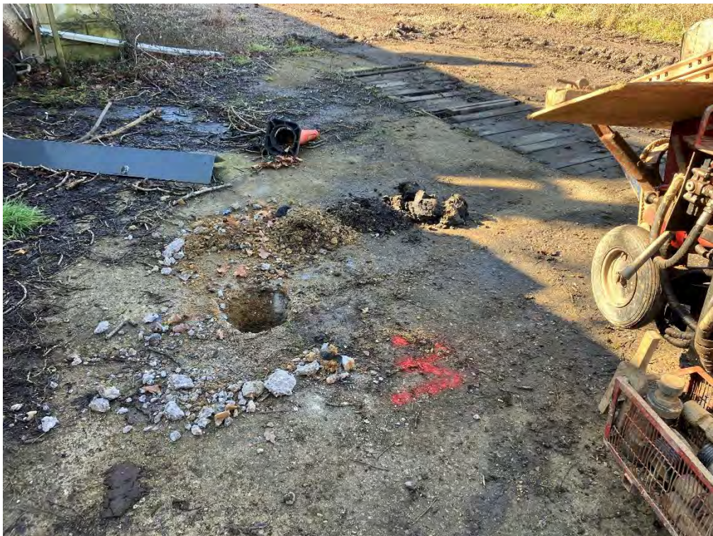
Equidistant position of borehole CT3 and excavated impacted near surface soils
