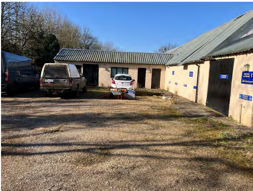
View from the entrance of Evendons Business Centre looking westwards (CT2)
