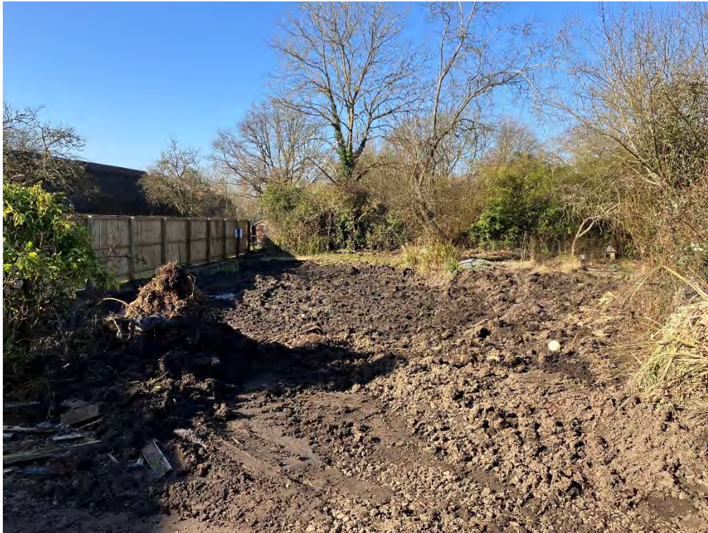
View of the recently backfilled pond (inaccessible) and foot access to western site area
