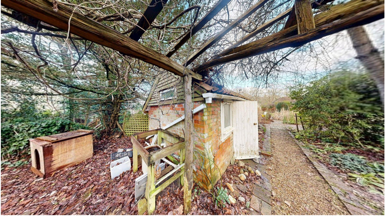
Outbuilding South West Elevation
