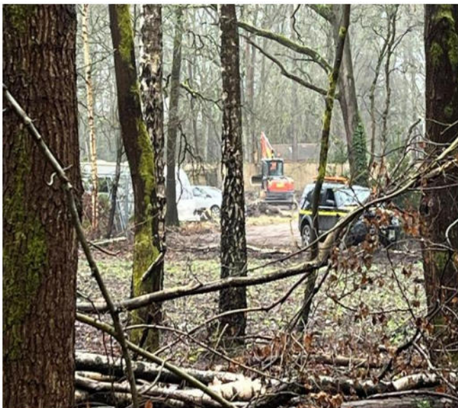
Figure 1: This was taken at 10.56 am on 7 th March 2026. There was not yet a static caravan and the works were still ongoing – the development was not complete.
