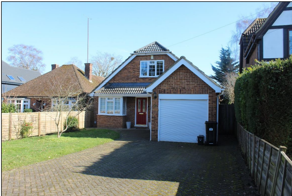
Photograph 1 – Front elevation as viewed from Nash Grove Lane
