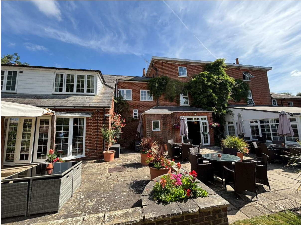
Part Rear Elevation of the Mill House Hotel taken from the private garden.
