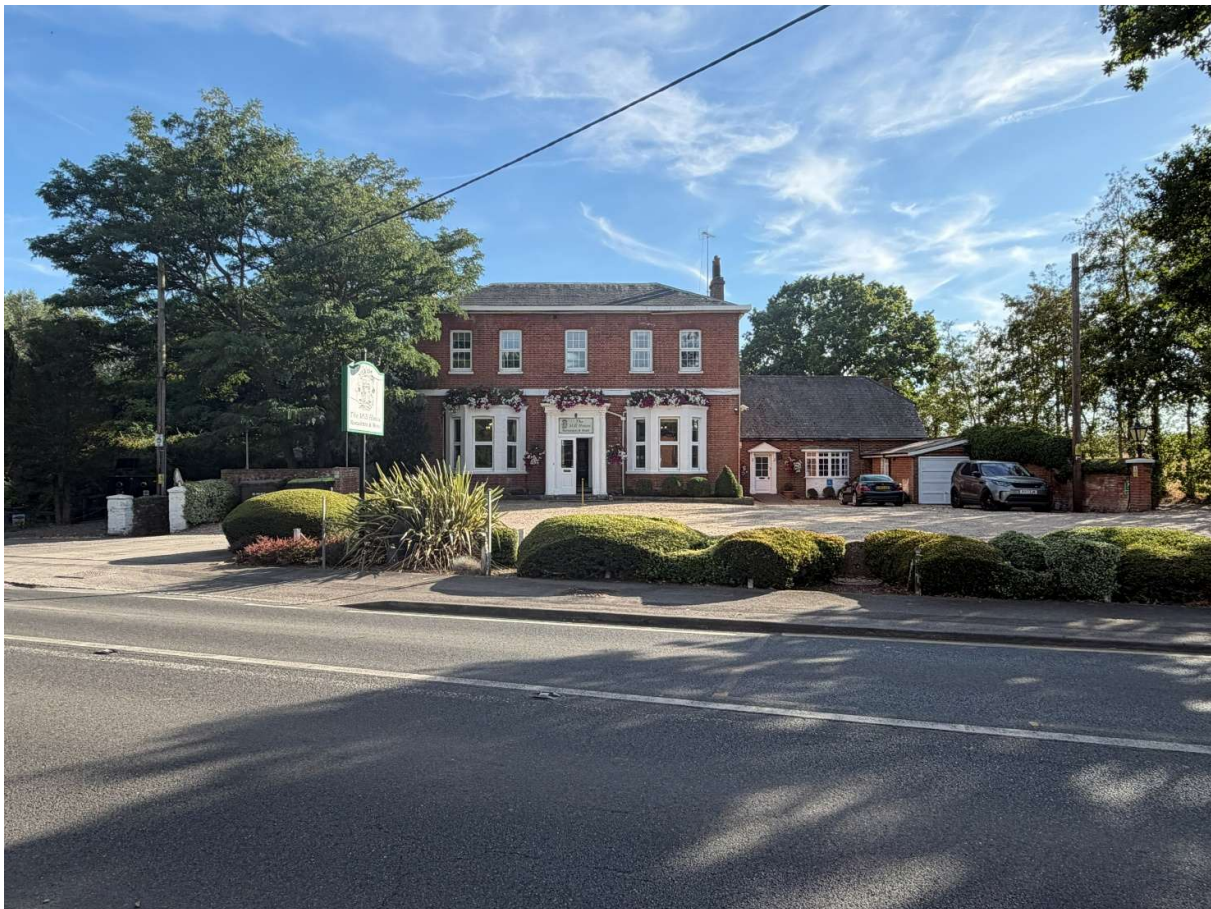
Front Elevation of the Mill House Hotel taken from the Basingstoke Road
