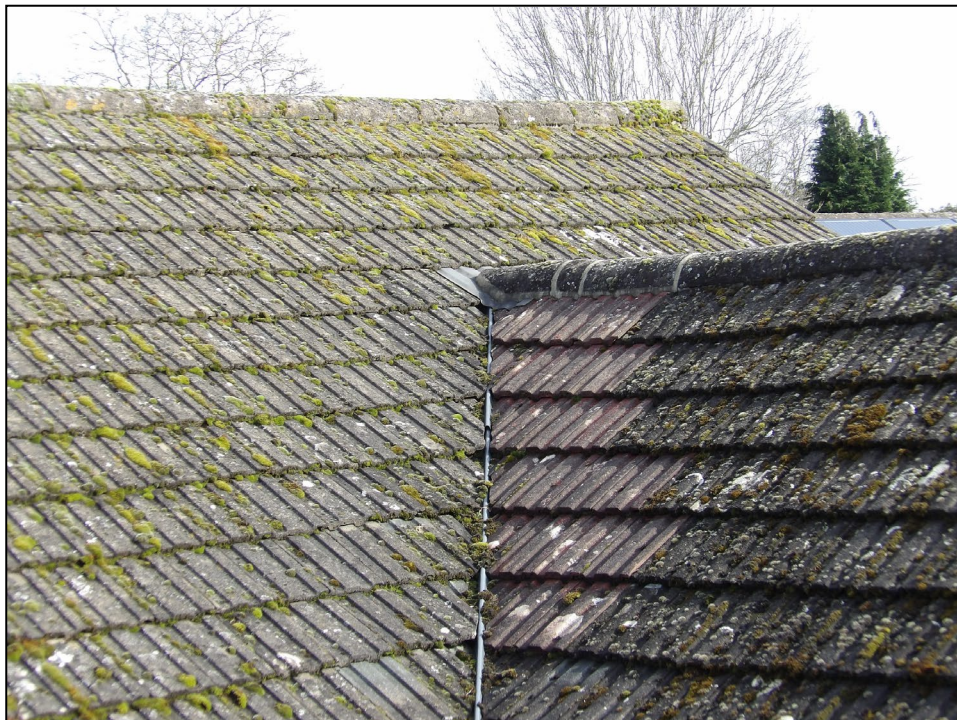
Figure 4. Example of sealed roof/ridge tiles and valley. 3 Northbury Avenue, Ruscombe. 25.02.25
