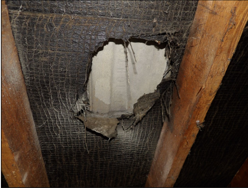
Figure 12. Example of ripped bitumen lining. 3 Northbury Avenue, Ruscombe. 25.02.25
