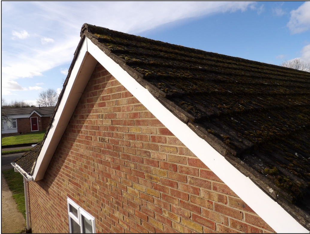
Figure 6. Example of soffits/fascias. 3 Northbury Avenue, Ruscombe. 25.02.25
