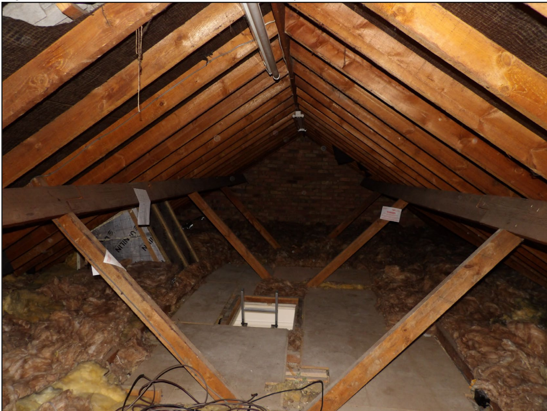
Figure 11. Example of loft space. 3 Northbury Avenue, Ruscombe. 25.02.25
