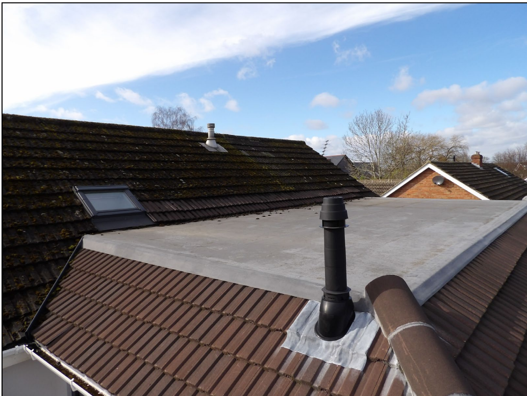
Figure 8. Rear extension. 3 Northbury Avenue, Ruscombe. 25.02.25
