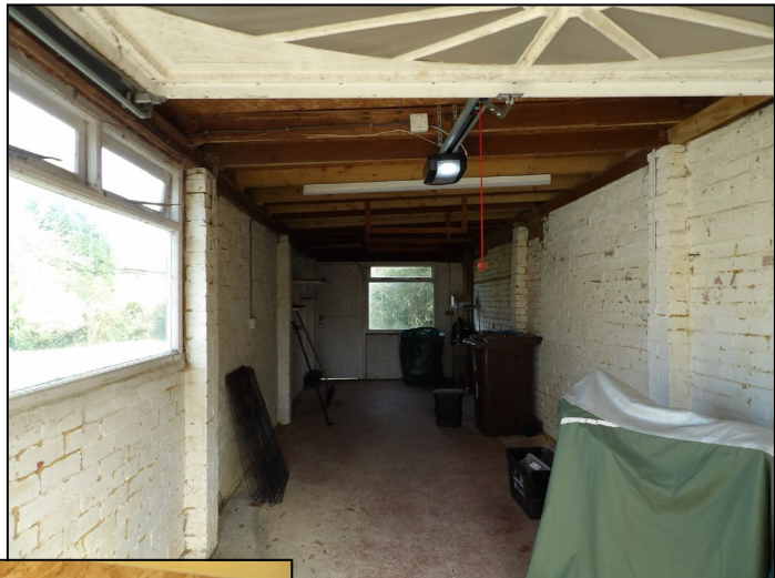
Figure 13. Internal view of garage and boarded ceiling. 3 Northbury Avenue, Ruscombe. 25.02.25
