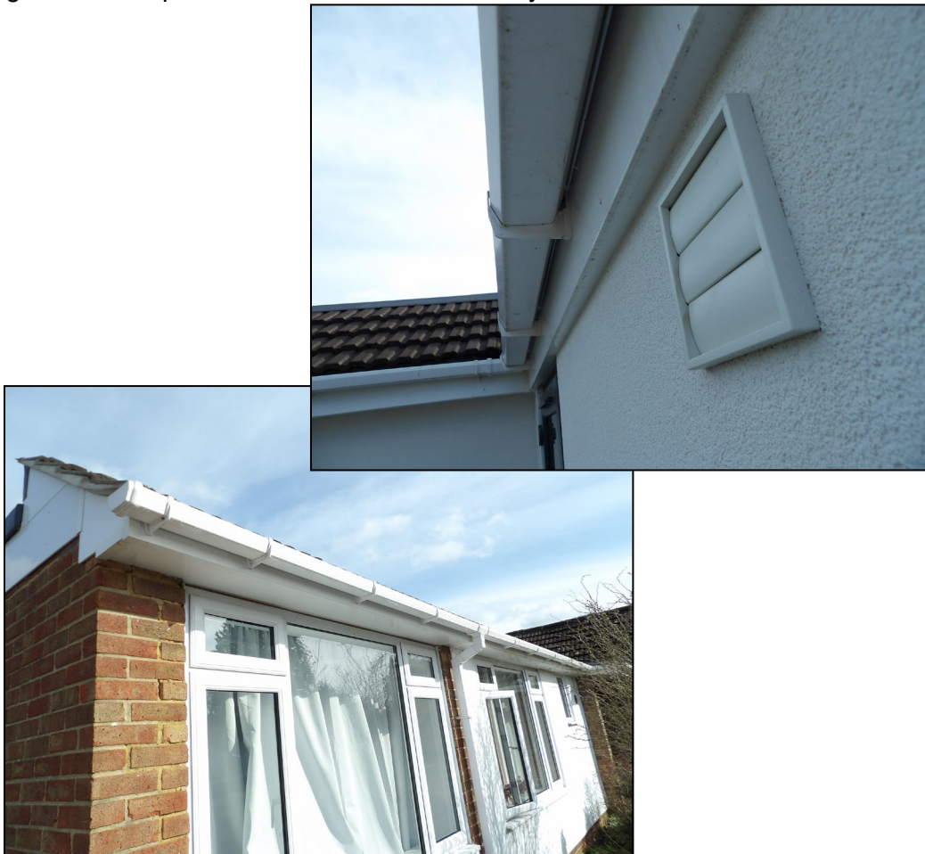
Figure 6. Example of soffits/fascias. 3 Northbury Avenue, Ruscombe. 25.02.25
