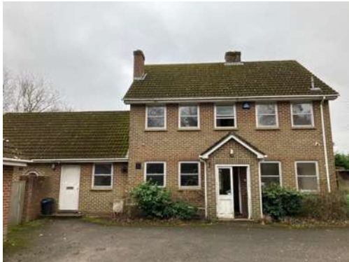
Photograph 1: B1, northern elevation
