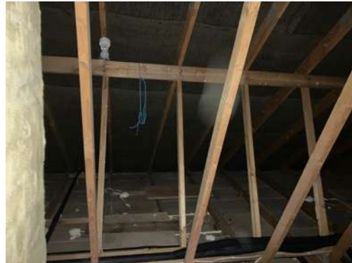
Photograph 2: Interior of B1
