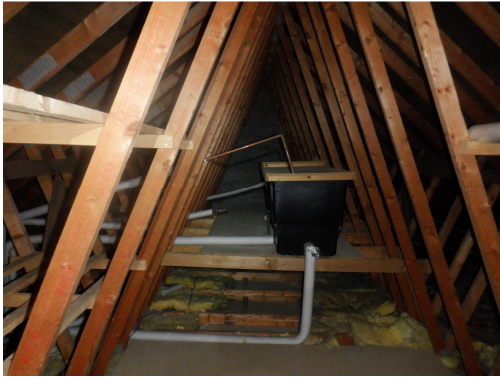
Photograph 13. Roof void of trussed construction.
