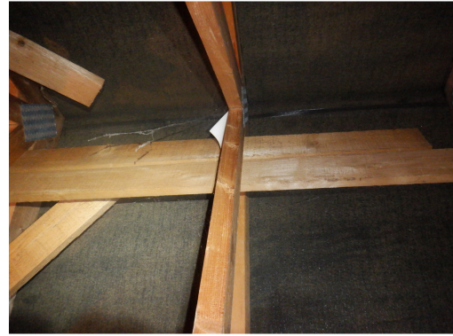
Photograph 14. Lightly cobwebbed ridge & fully intact bitumen felt (roof void).
