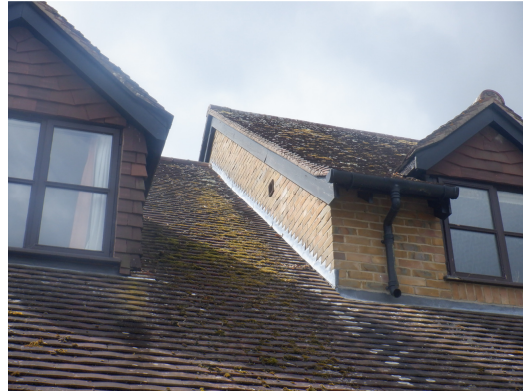
Photograph 6. Lead flashing sealed along the dormer windows and roof of the half-hipped extension (front elevation).
