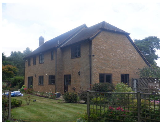
Photograph 2. Rear and side of property viewed from the southeast.
