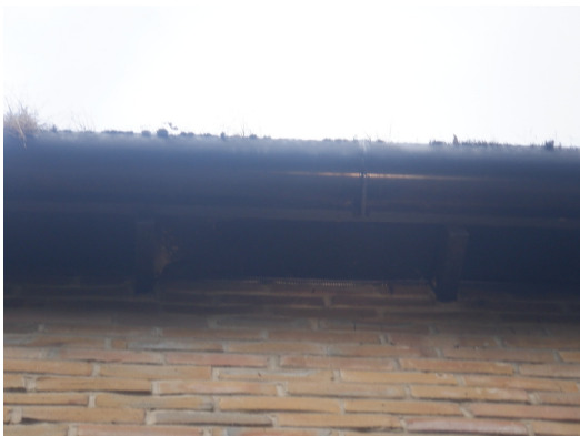
Photograph 7. Eaves fully sealed (rear elevation).
