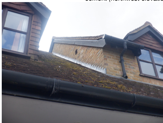
Photograph 9. Timber fascia sealed to gable (front elevation).
