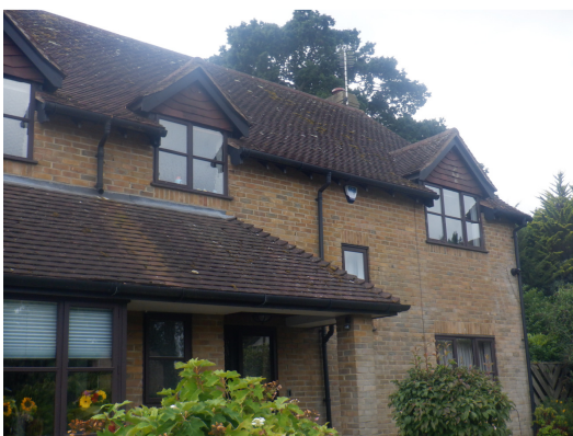
Photograph 1. Front of property viewed from the northeast.
