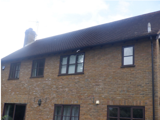
Photograph 5. Lead flashing sealed to chimney and roof tiles (rear elevation).
