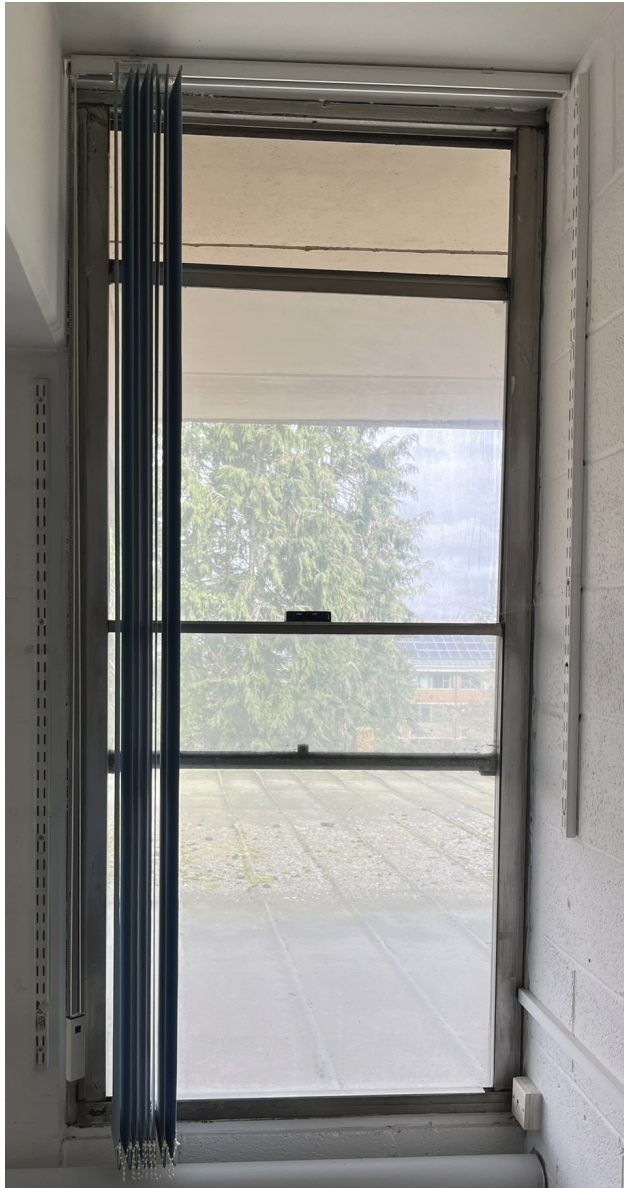
Existing sliding sash window (Level 3)
