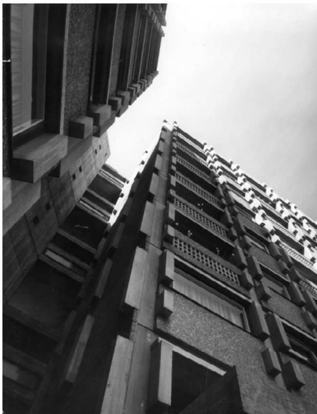
Weston Rise Housing Estate, Islington. Photographed 1969 by Henk Snoek (RIBA, RIBA26194, Permission pending)
