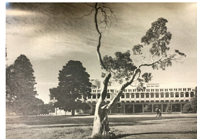
North elevation of the URS building, looking across the open greensward (AR, November 1973, p. 279)
