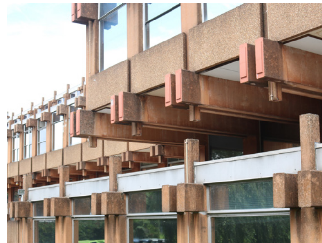
Standard beams (below) and post-tensioned beams, distinguished by the infilled anchorage pockets (above)
