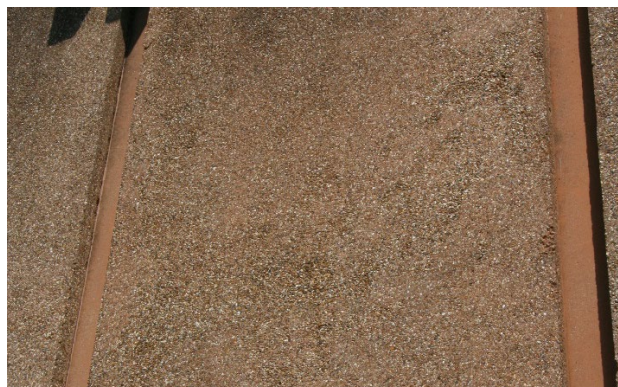
Example of Defect Type B7
