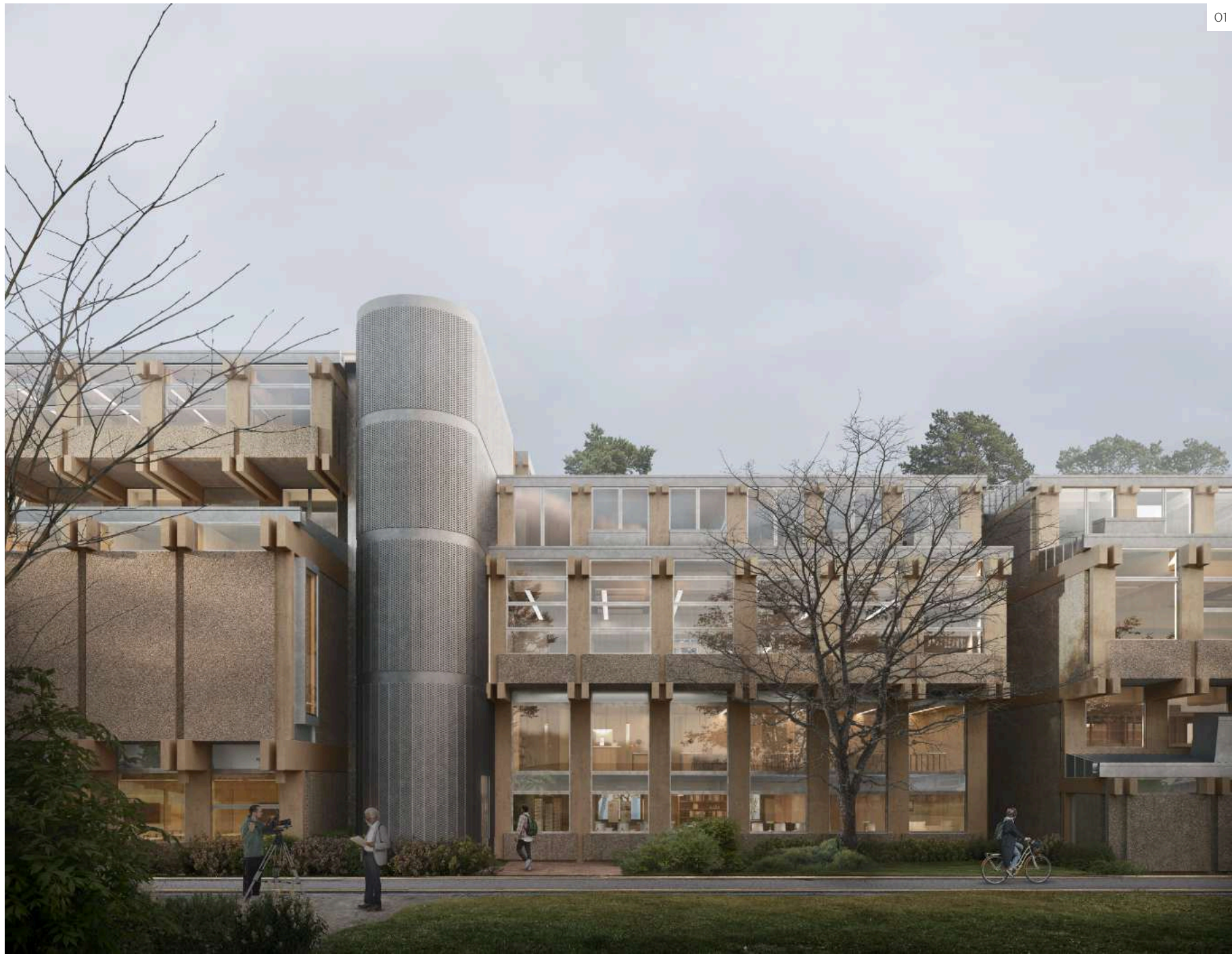
01 Exterior image of the southern facade of the URS Building.
