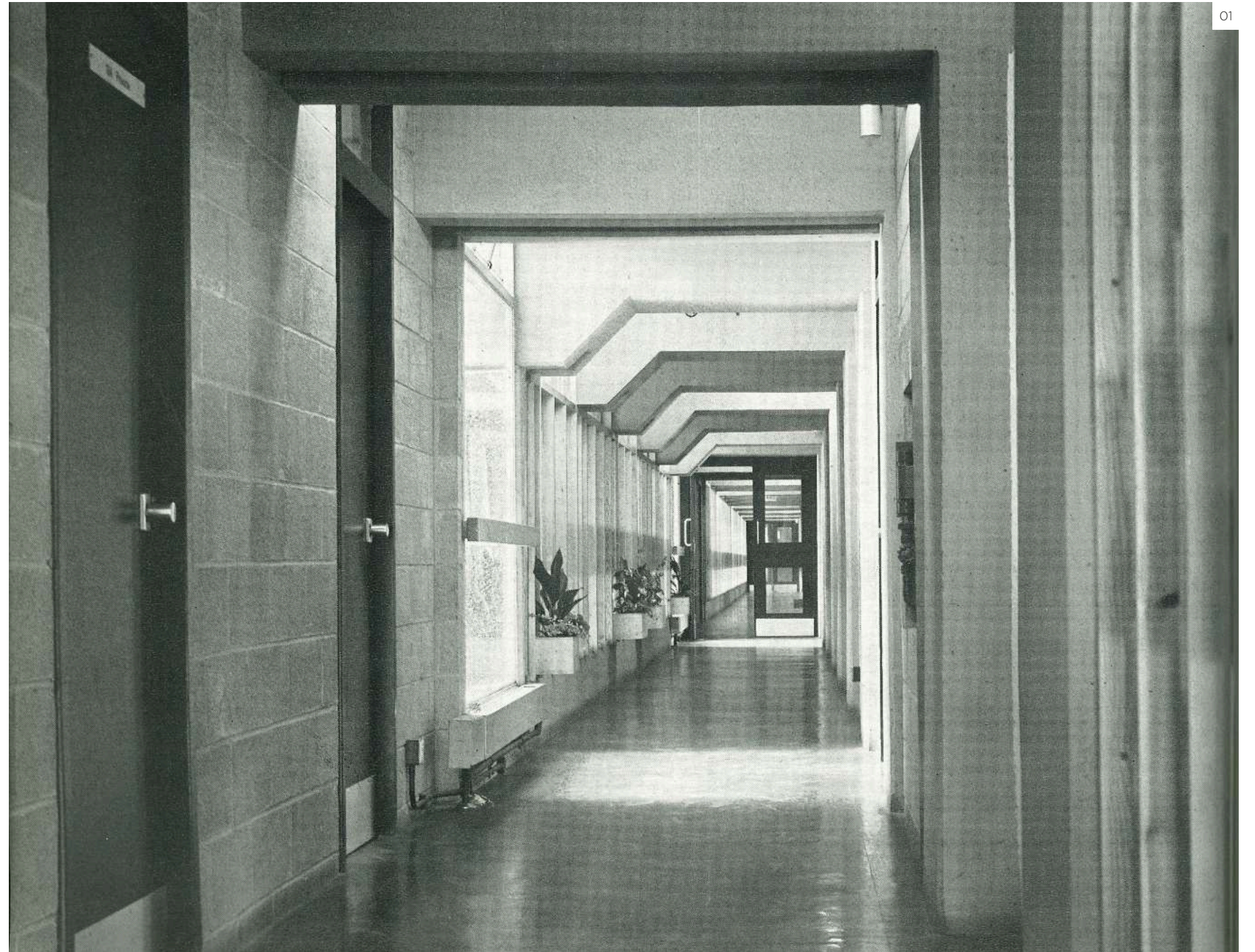
01 Photo of original URS first floor corridor, taken from the November 1973 edition of the Architectural Review.
