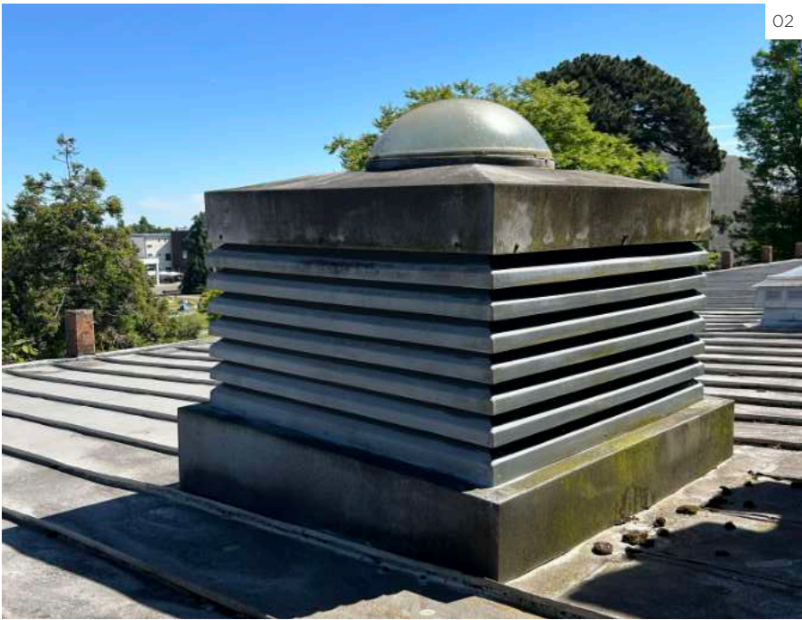
01 Indicative 3D model of proposed cowls. 02 Existing roof cowl. 03 Precedent image of proposed roof cowl.
