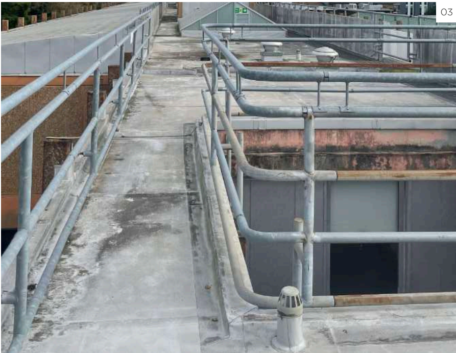
01 Image of the original roof handrail system, taken from the November 1973 issue of the Architectural Review magazine. 02 Image of the original roof handrail system, taken from the November 1973 issue of the Architectural Review magazine.
