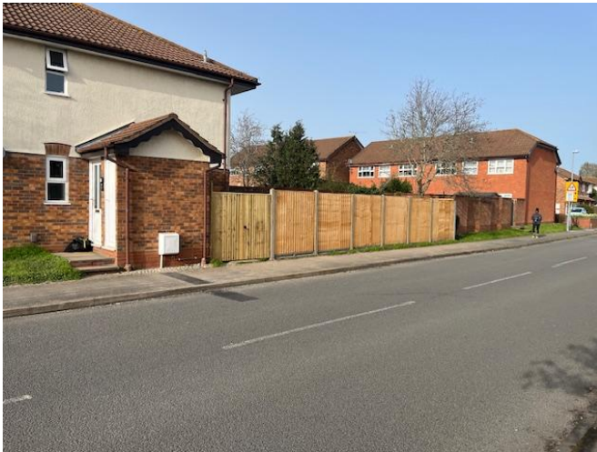
Fence at 9 Hurricane Way. Photo taken from southwest looking northeast.
