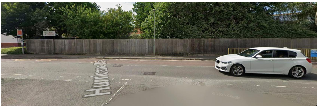
Wooden fence fronting Hurricane Way viewed from Comet Way. To the east of the application site.
