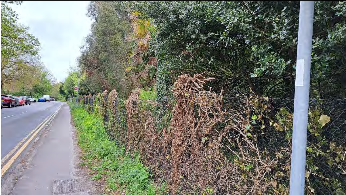
Vegetation and existing fence along edge of Harris Garden at southern end of Site.
