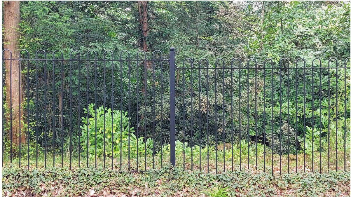
Above: Photo of existing fence at Whiteknights Road. This is to be retained, and new fences shall visually match.
