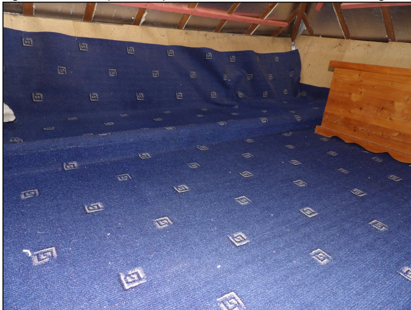
Figure 11. Example loft space. 46 Bearwood Road, Wokingham. 08.04.25
