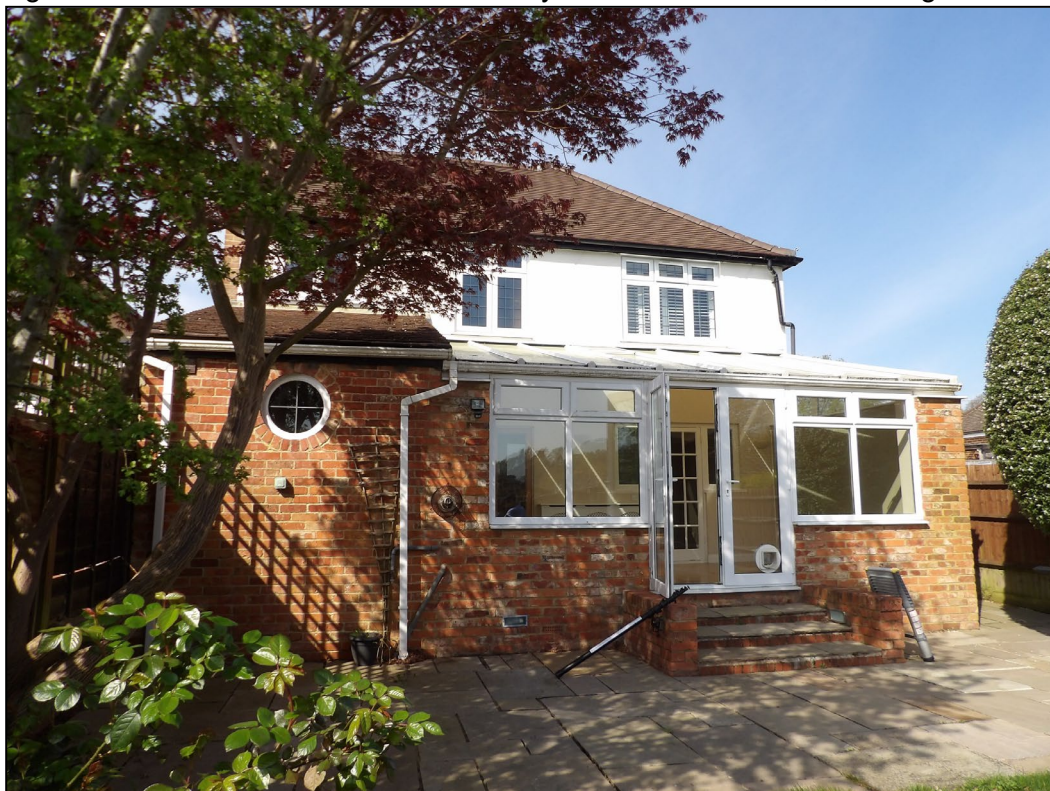
Figure 8. Rear extension and conservatory. 46 Bearwood Road, Wokingham. 08.04.25
