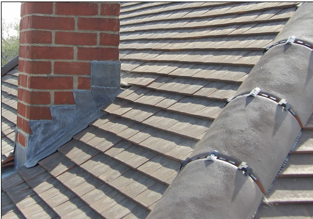
Figure 6. Example of lead flashing. 46 Bearwood Road, Wokingham. 08.04.25
