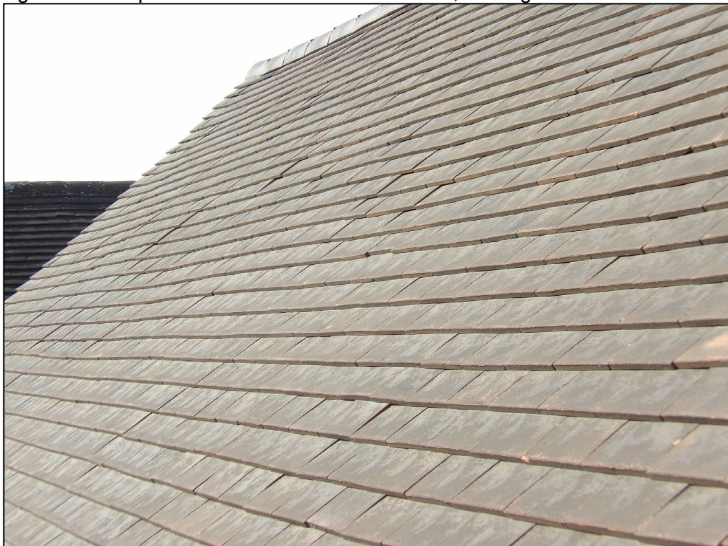
Figure 4. Example of roof tiles. 46 Bearwood Road, Wokingham. 08.04.25
