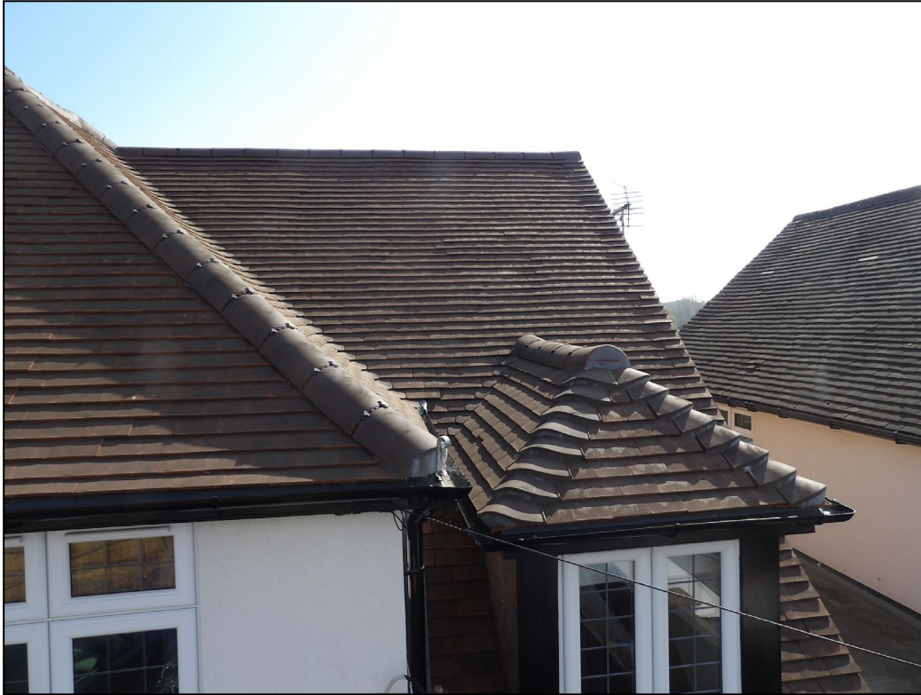
Figure 5. Example sealed ridge and hips tiles. 46 Bearwood Road, Wokingham. 08.04.25
