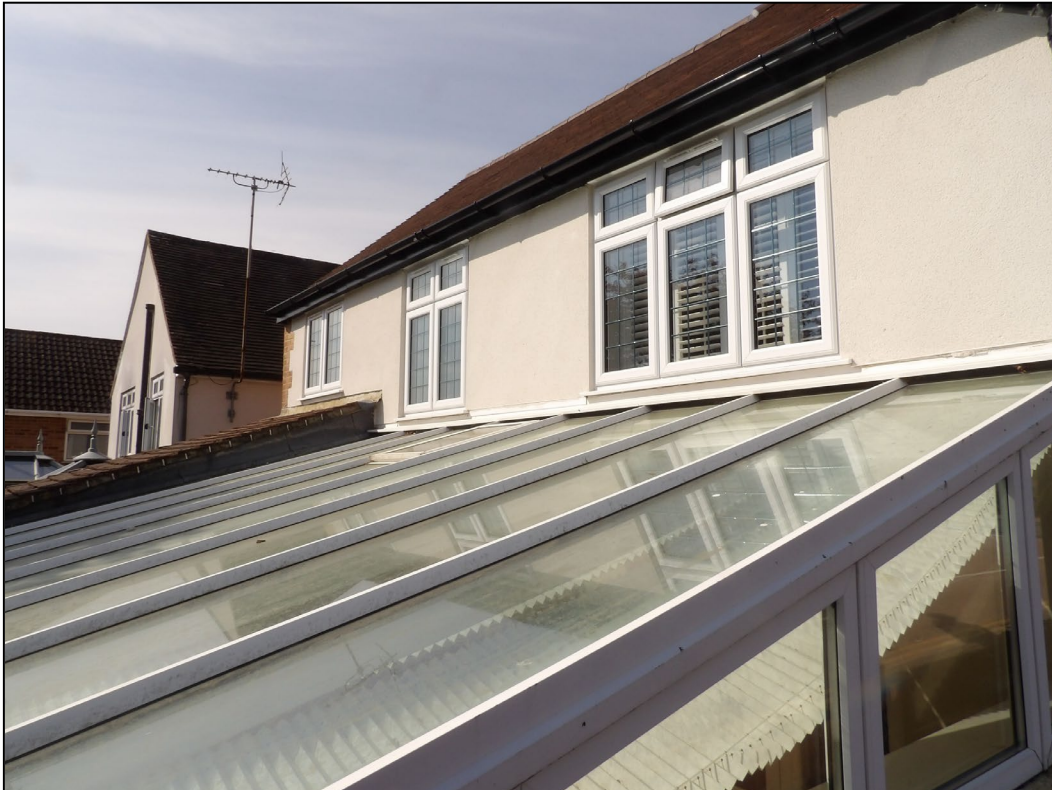
Figure 10. Glass roof of conservatory. 46 Bearwood Road, Wokingham. 08.04.25
