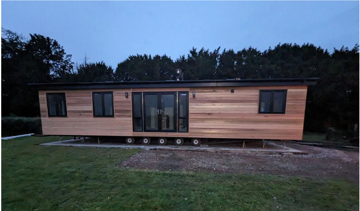
APPENDIX C IMAGE 01 – Example of home on a chassis on site with concrete pad 01
