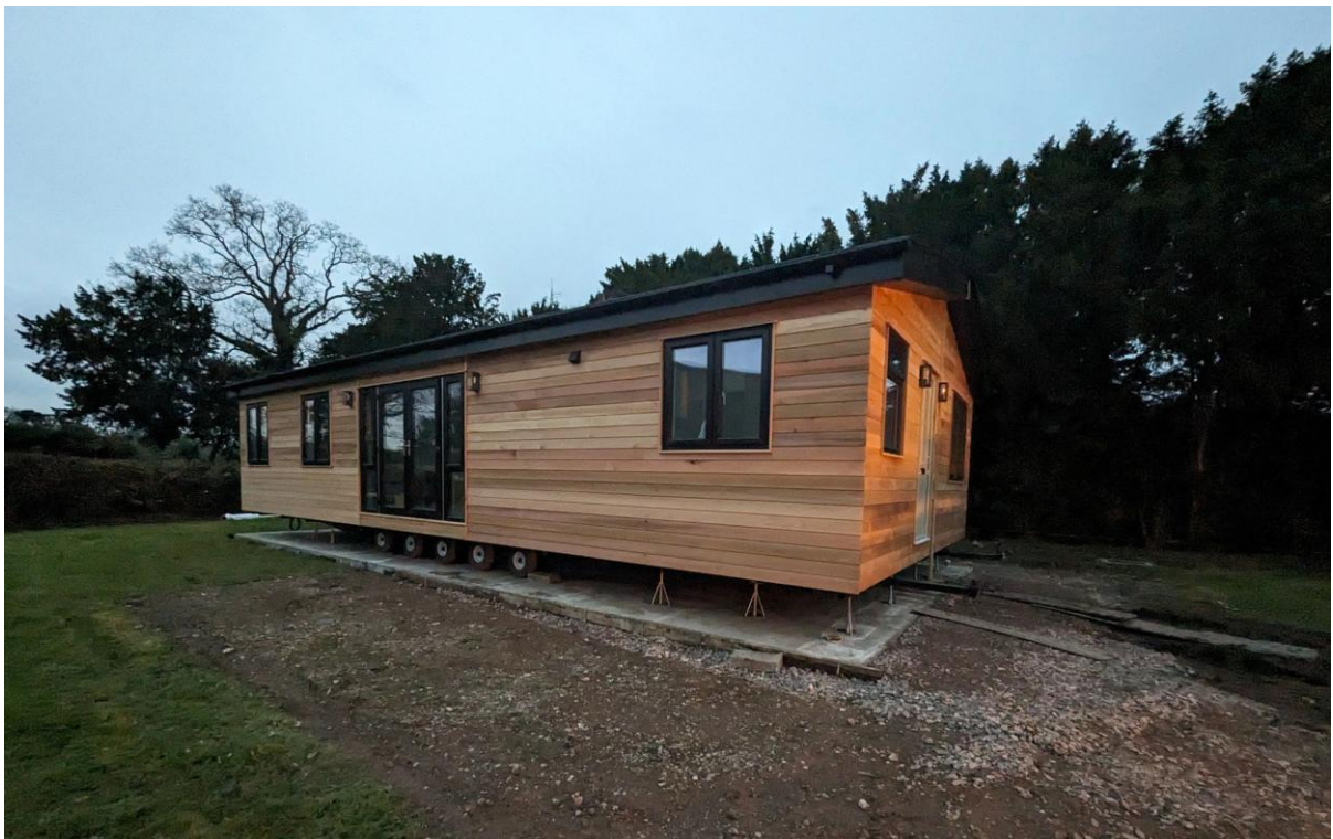
APPENDIX C IMAGE 02 – Example of home on a chassis on site with concrete pad 02
