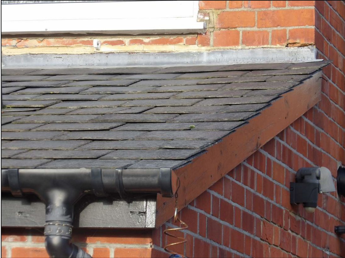
Figure 5. Example of slate roof tiles. 45 Hatch Ride, Crowthorne. 03.12.24
