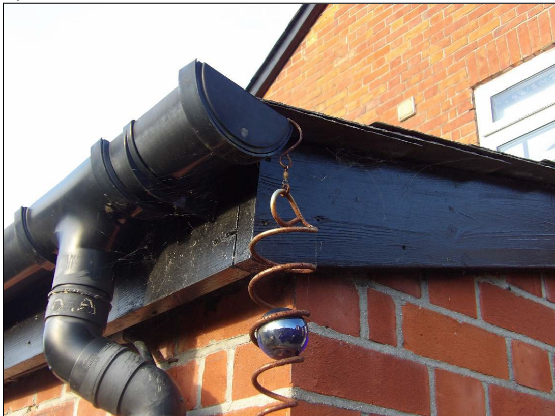
Figure 6. Soffits and fascias. 45 Hatch Ride, Crowthorne. 03.12.24
