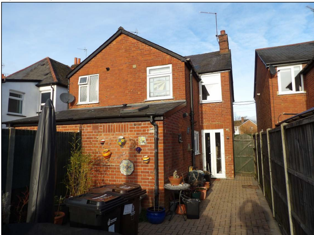
Figure 4. Single storey rear extension. 45 Hatch Ride, Crowthorne. 03.12.24
