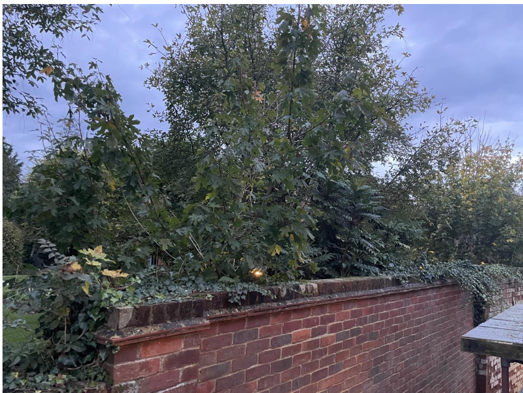
Figures 2- 3: Site photos (Oct 2024) illustrating brick boundary wall and adjacent trees in the Remeneham Row estate
