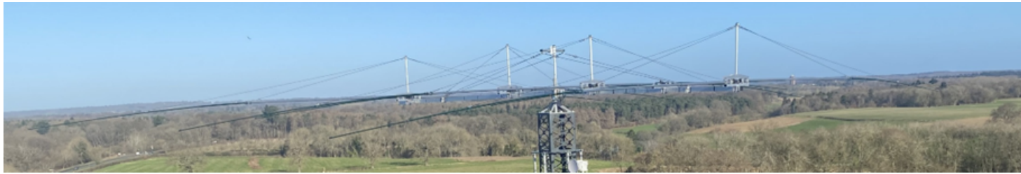
Example photograph of similar boom and antennae arrangement
