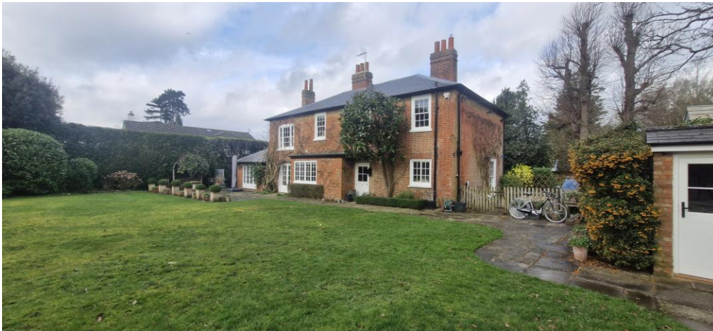
Photo 6: Rear elevation of the property
