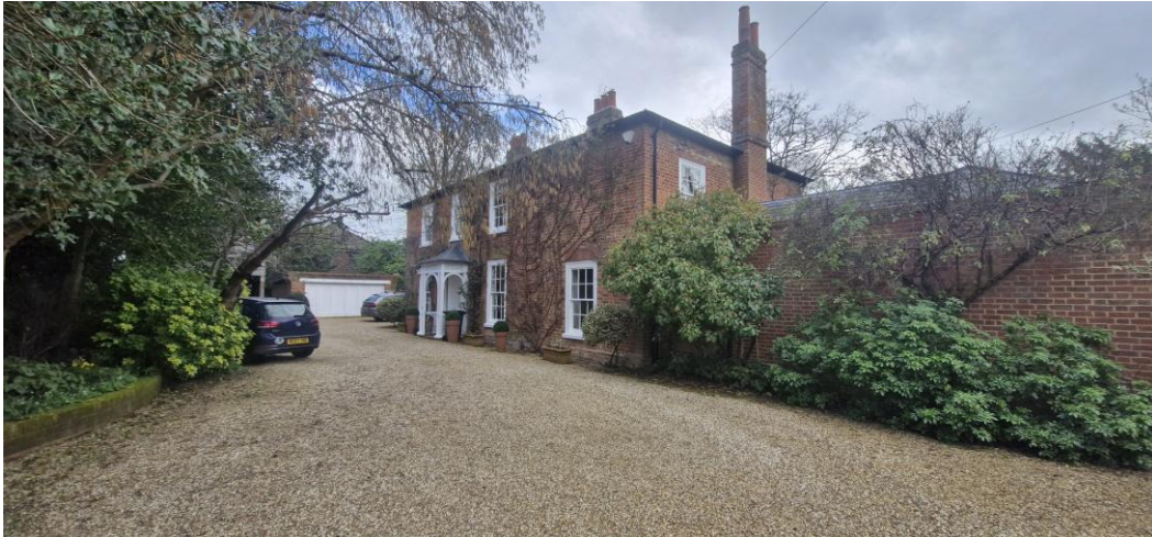
Photo 5: Front elevation of the property
