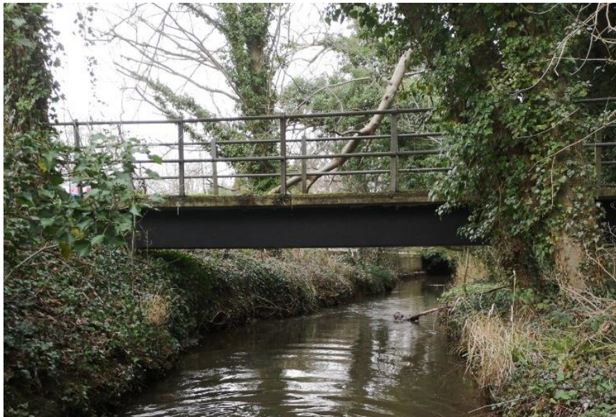
Figure 16 Un-named bridge across existing channel
