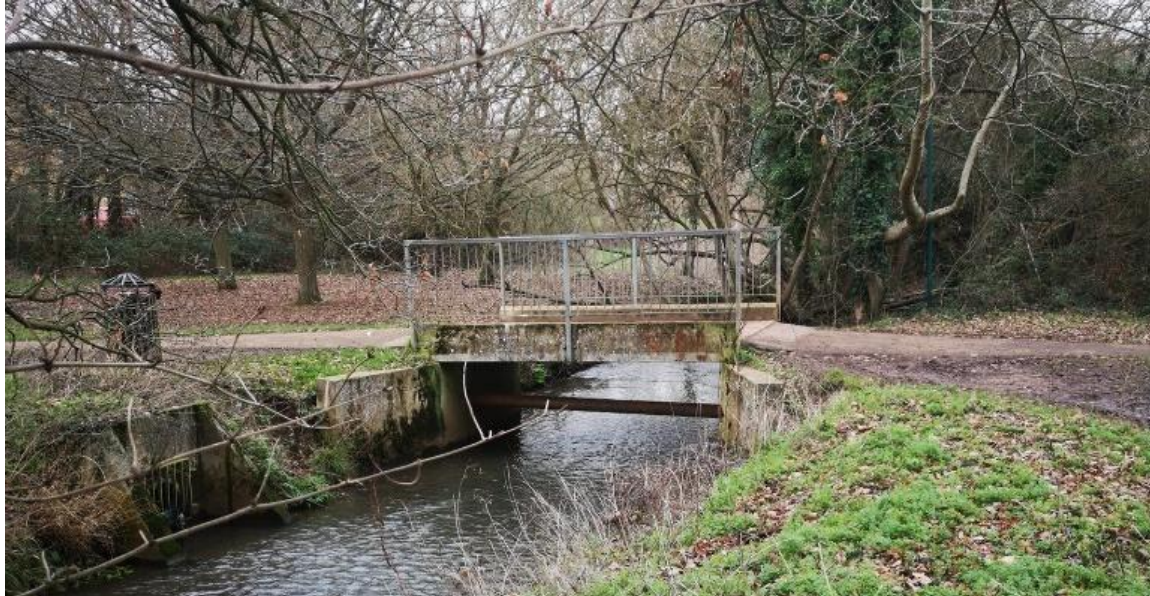
Figure 15 Kingfisher bridge, existing channel. Note that the pipe obstruction beneath the bridge is also modelled.
