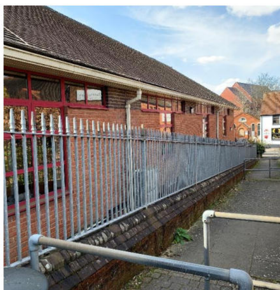
Photo 05: External Ramp Access and North Elevation
