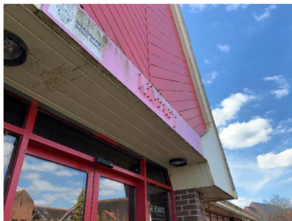
Photo 03: Existing North Entrance Door Soffit
