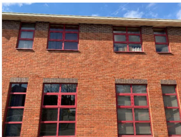
Photo 02: Existing East Elevation Windows
