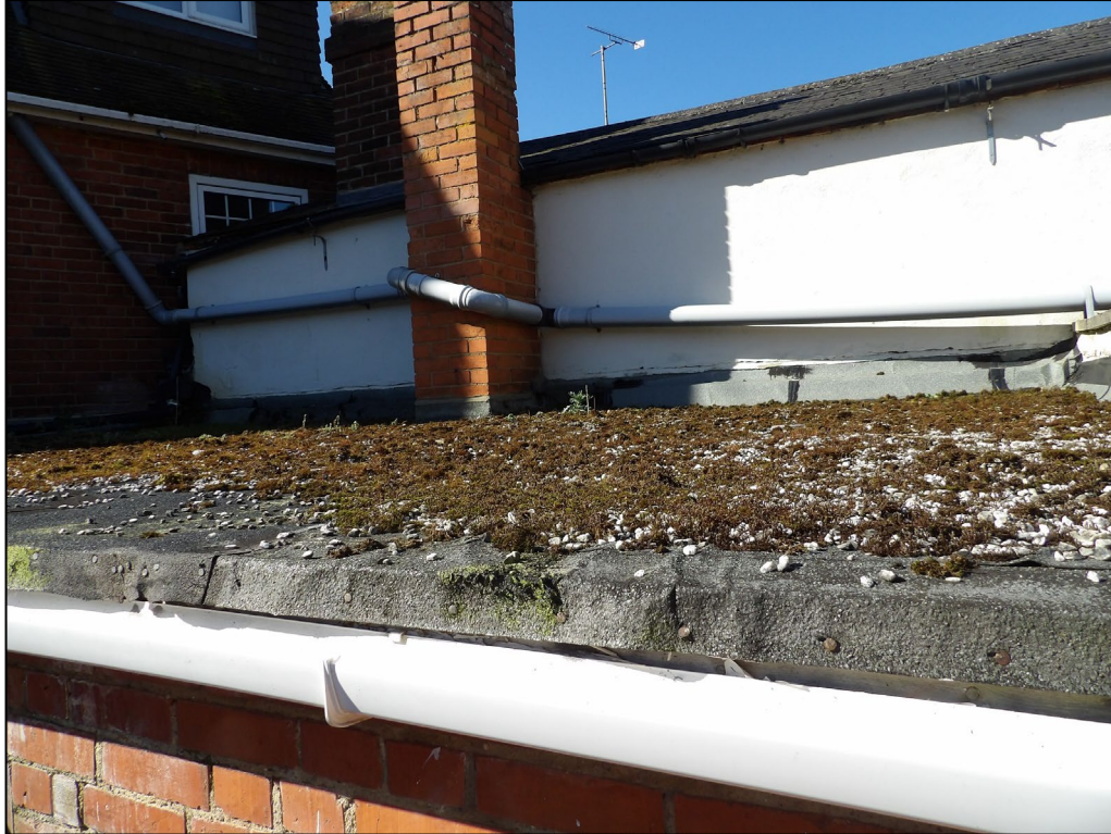
Figure 5. Example of bitumen covering on roof of rear extension. 56 High Street, Twyford. 18.03.25
