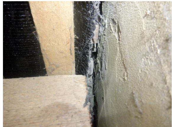
Photograph 14. Slight cobwebbed gap beside chimney, with underside of roof tiles visible (roof void).
