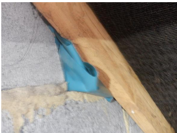
Photograph 15. Plastic sheeting visible in gap over blockwork (roof void).
