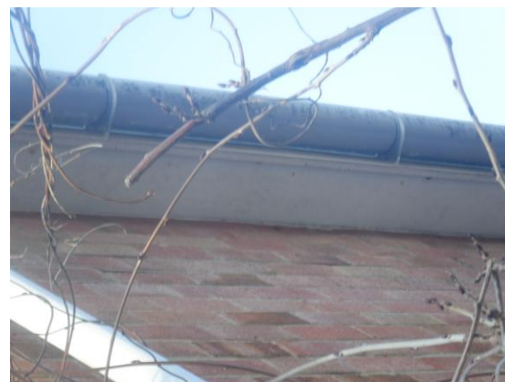
Photograph 6. Intact sealant along the eaves of the main roof (eastern elevation).
