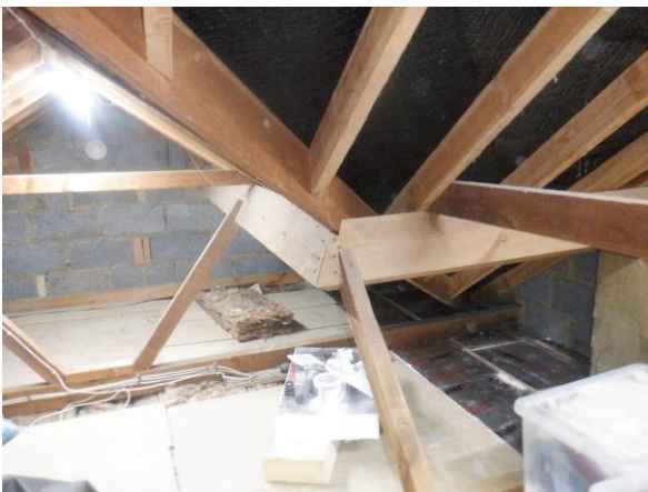
Photograph 9. Boarding and fibreglass insulation in the centre of the void and celotex insulation (roof void).
