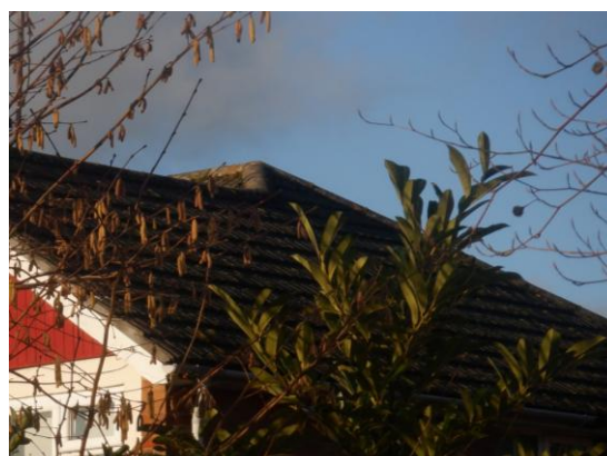
Photograph 4. Ridge and hip mortar intact (eastern elevation).
