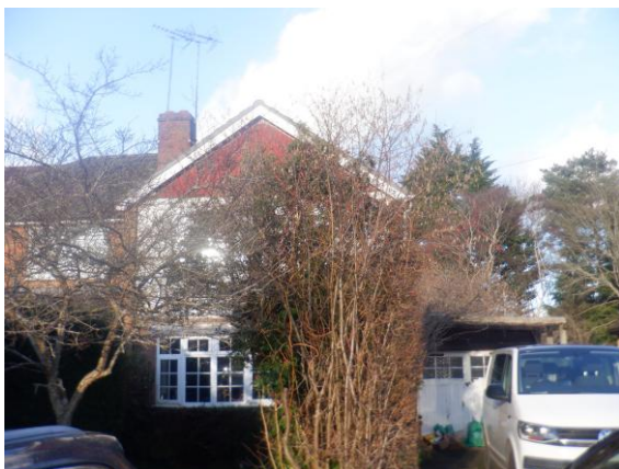
Photograph 1. Front of house viewed from south.
