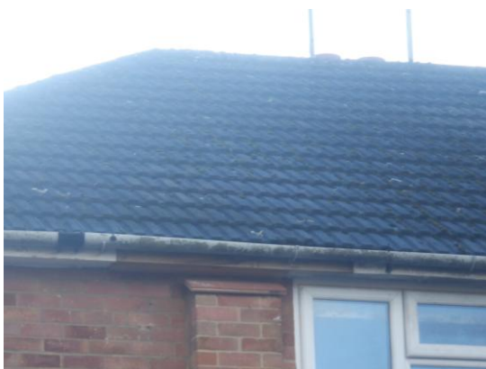
Photograph 3. Tight interlocking roof tiles (northern elevation).
