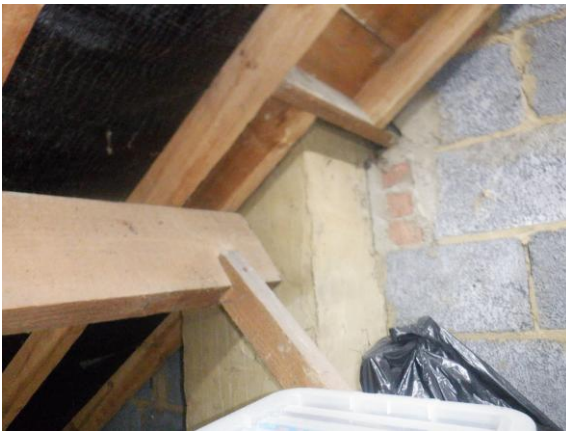
Photograph 13. Rendered chimney on the western party wall (roof void).
