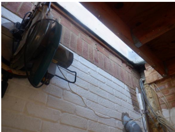
Photograph 16. Skylight in roof adjacent to the wall of the house (garage).
