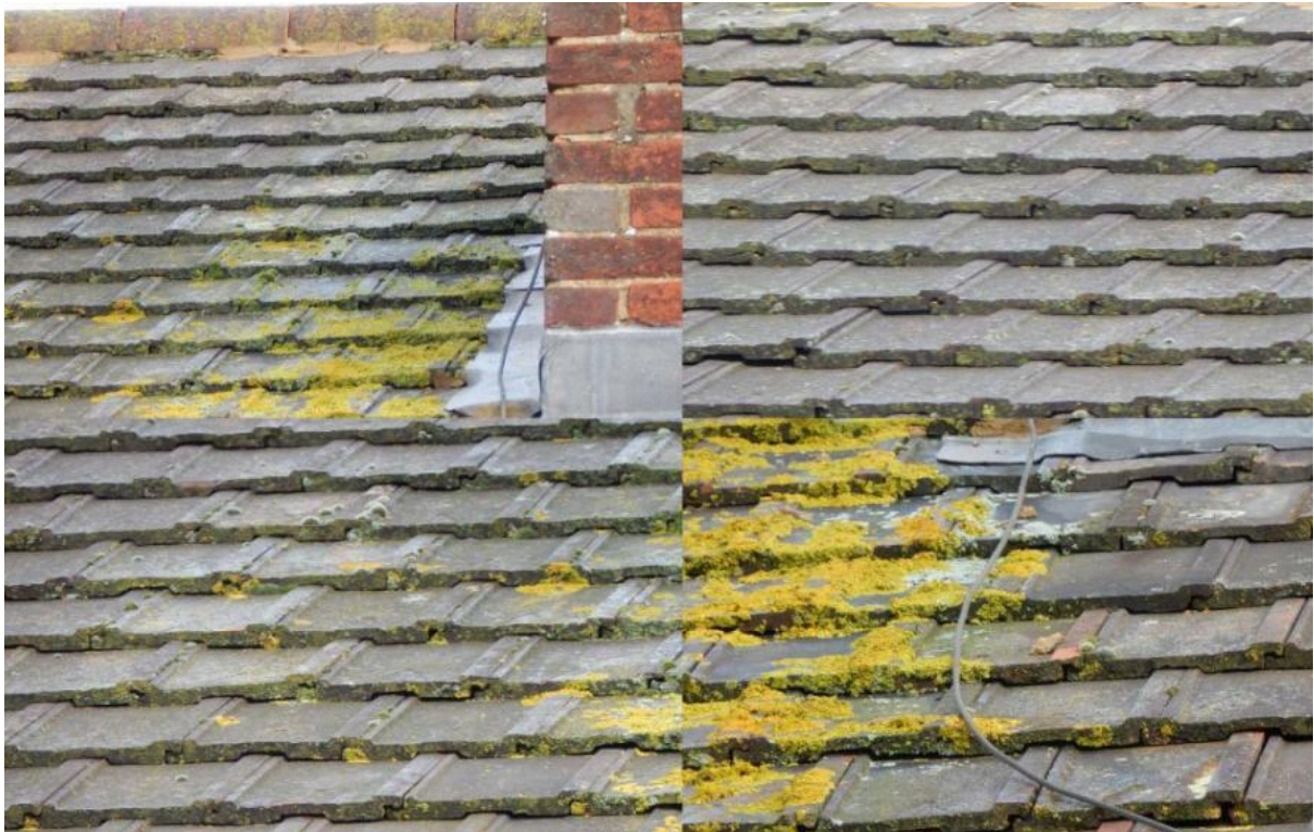
Image 5 – Close view of upper tiled roof coverings to demonstrate condition throughout
