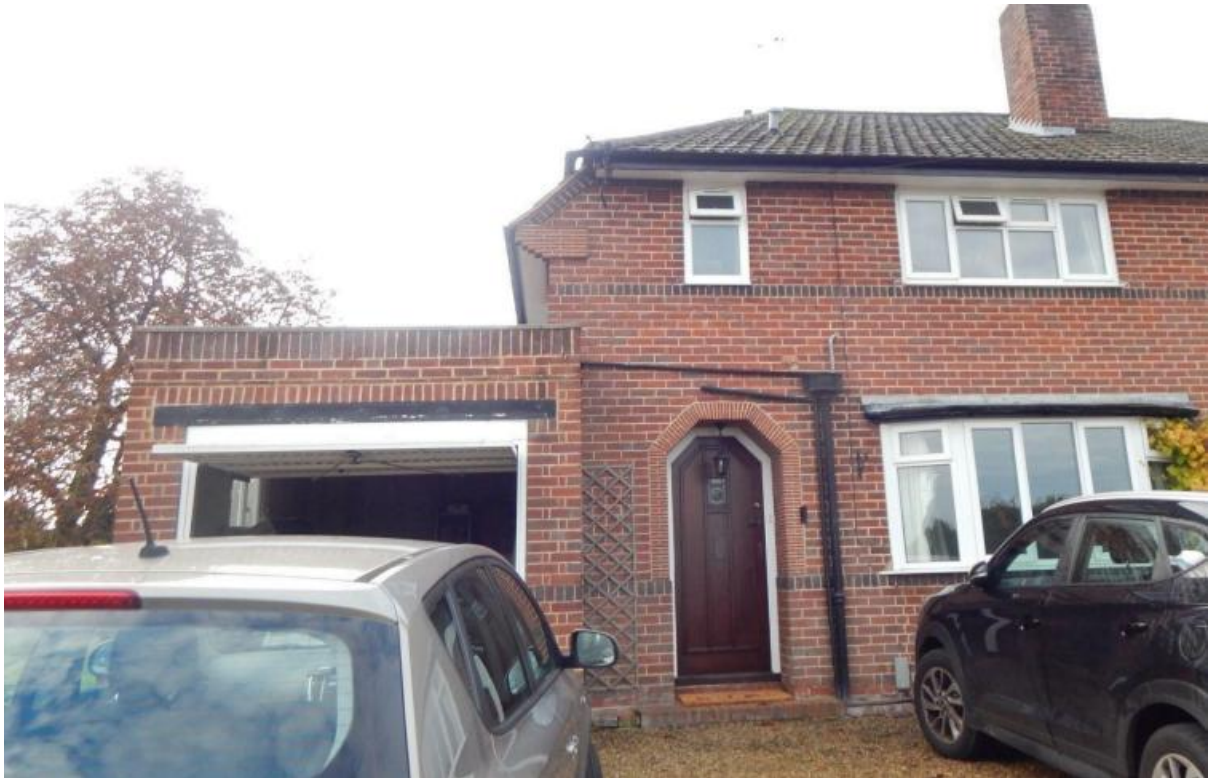
Image 1 – North facing elevation of the property
