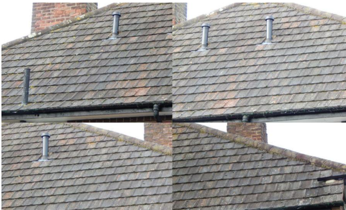
Image 4 – Close view of upper tiled roof coverings to demonstrate condition throughout
