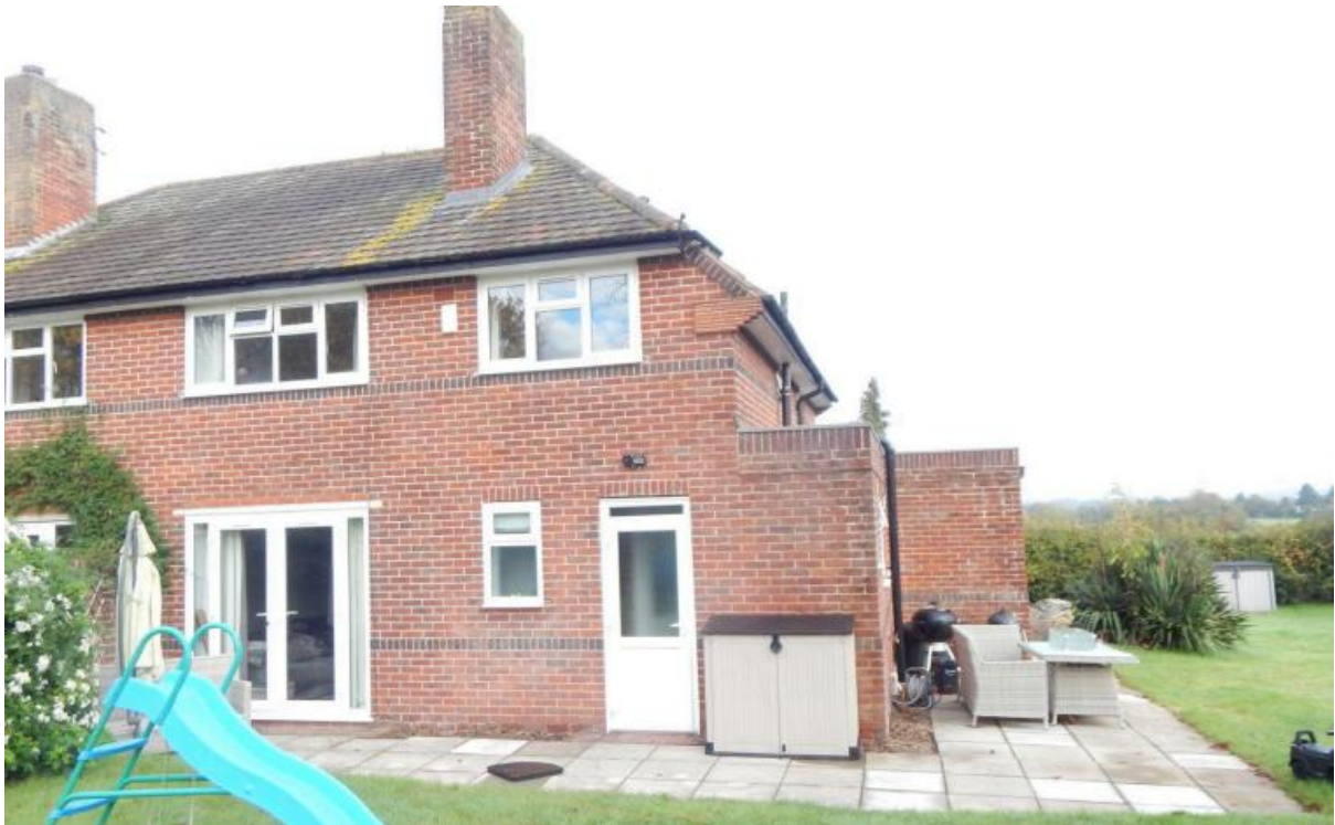
Image 2 – South facing elevation of the property
