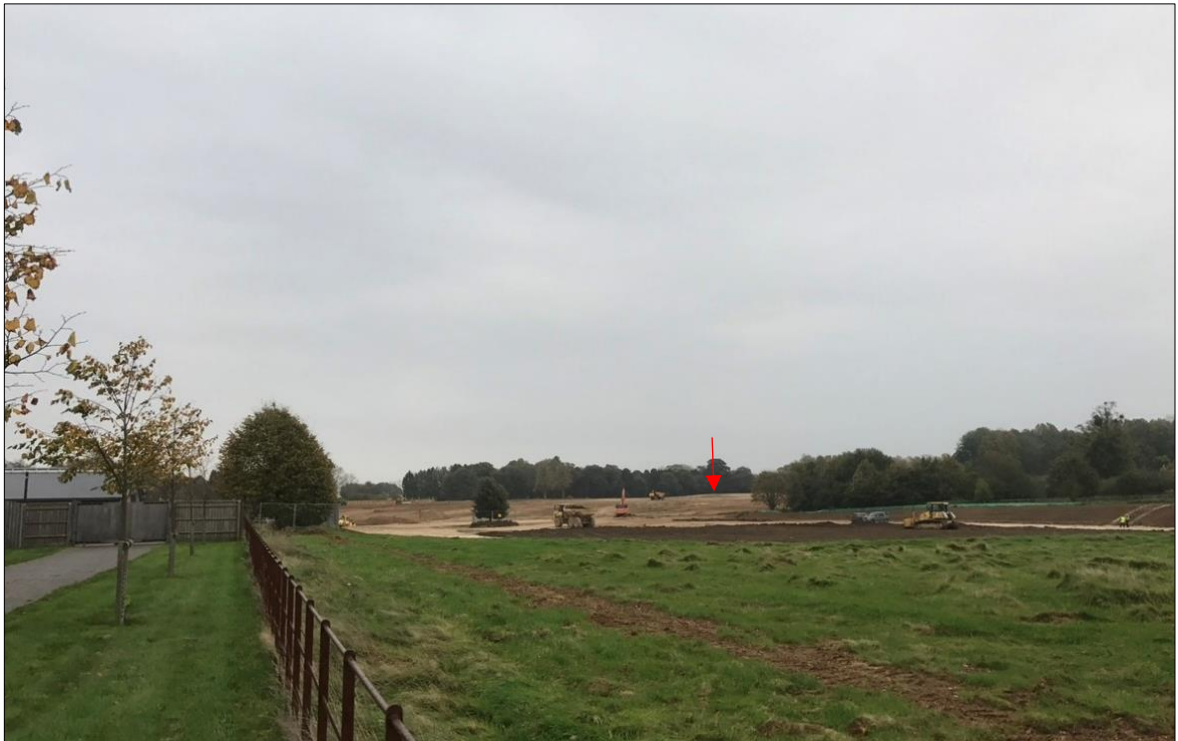
Fig. 6 – Photo taken by [REDACTED] (Polo Manager) 17 October 2017 showing the earth moving plant and vehicles on the site. The northern end of the viewing mound along the western edge of the polo pitch is visible (in the process of construction).
