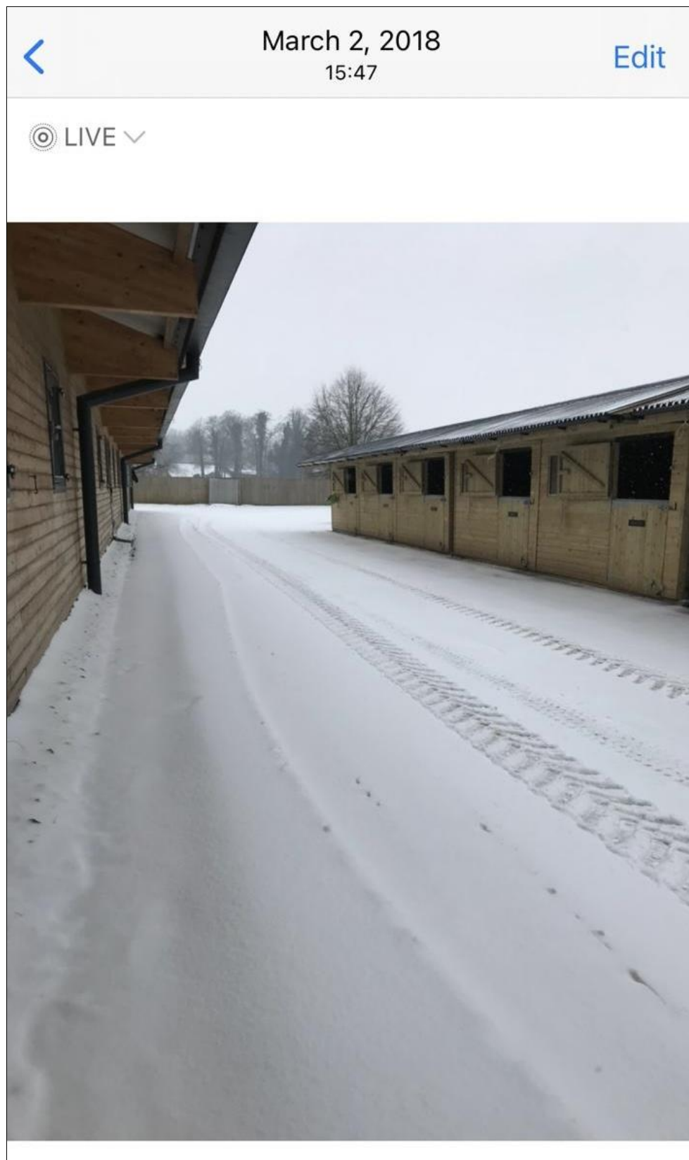
Photo. 4 – Shows the row of stable buildings on the western side of the American barn
