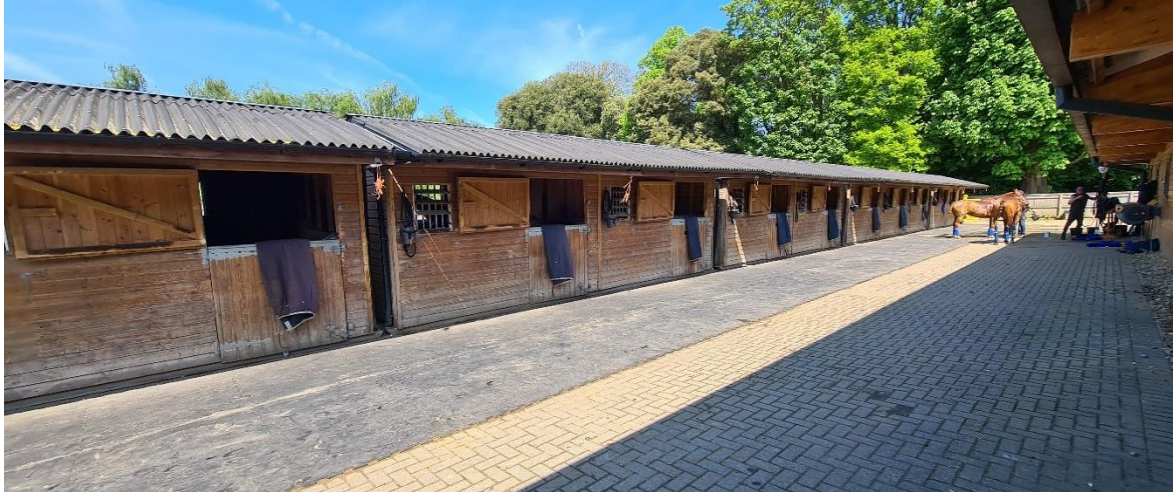
Fig. 2 - Row of stable buildings on the western side of American barn (May 2024)
