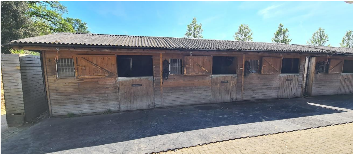
Fig. 3 – Stable buildings on the eastern side of American Barn; triple unit shown (May 2023)
