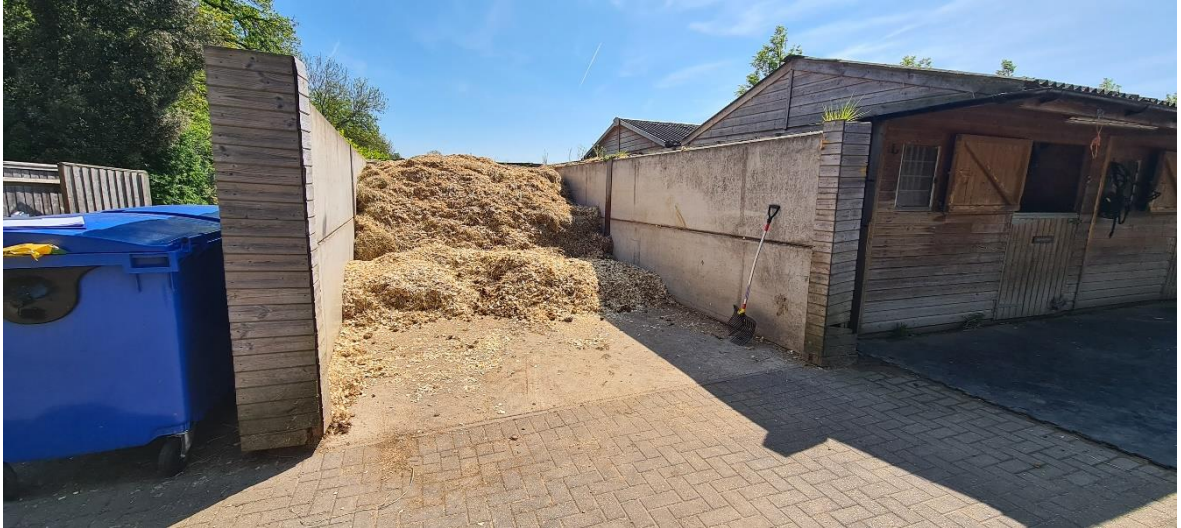
Fig. 7 – Muck heap enclosure (May 2024)
