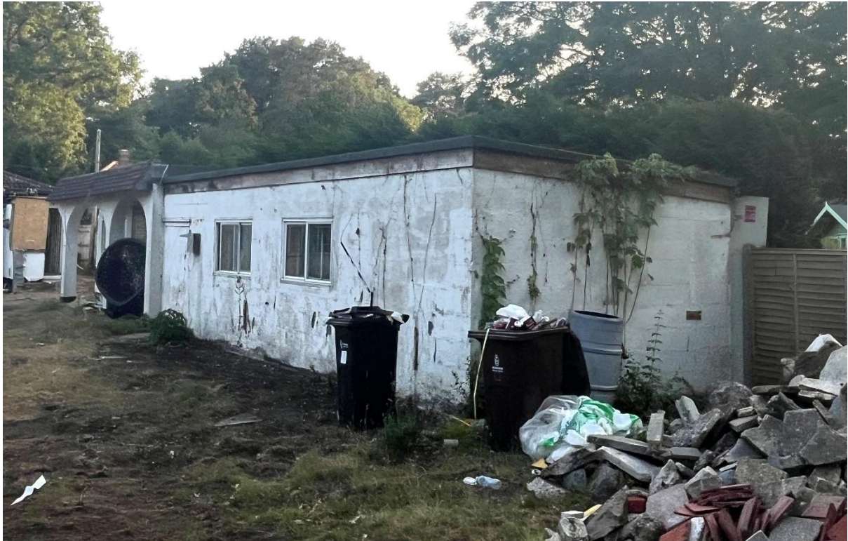
Figure 6. Rear extension looking southwest.
