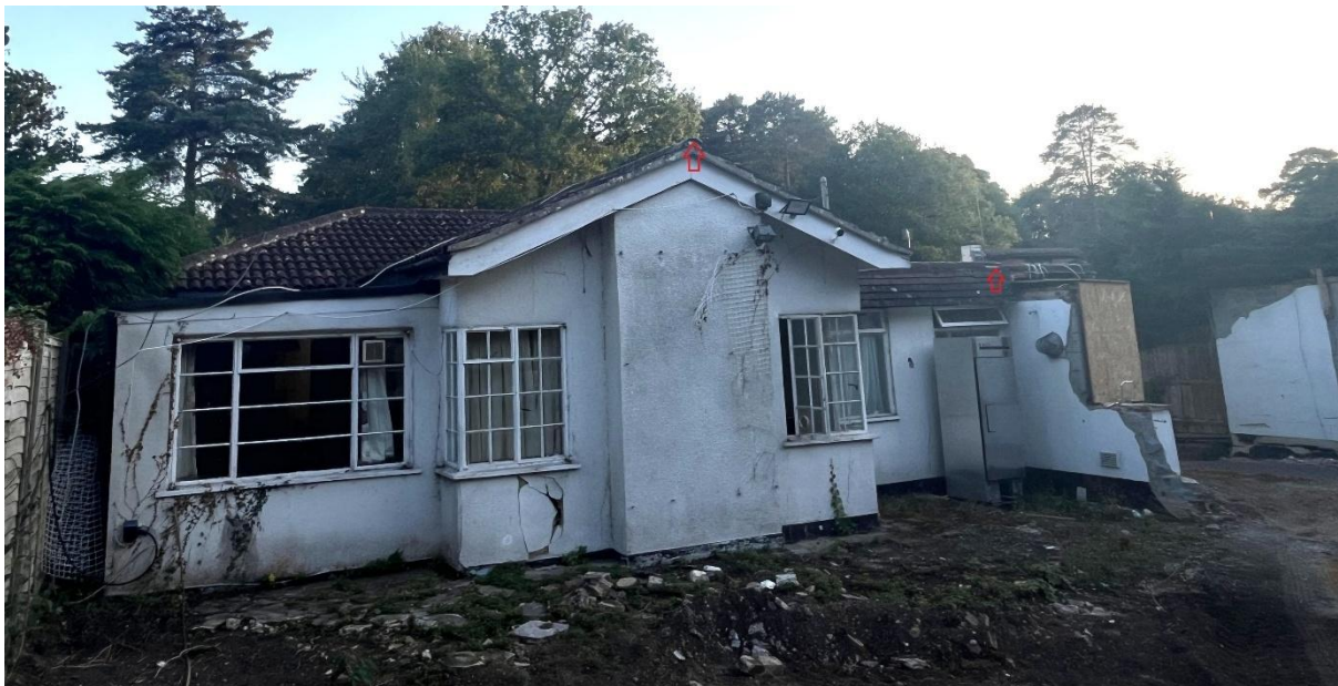
Figure 4. Rear elevation of bungalow looking southwest: Red arrows indicate potential openings for crevice roosting bats.
