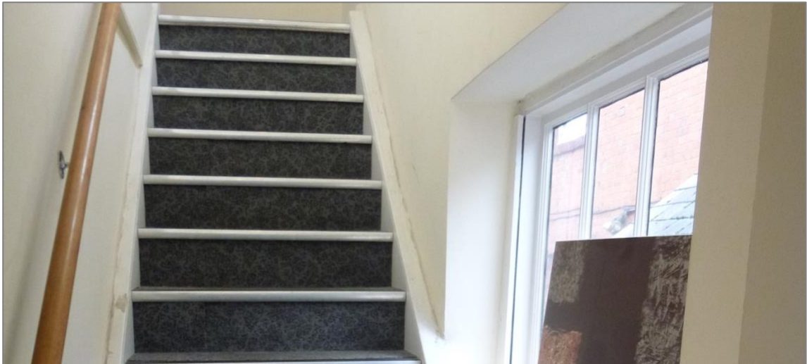
Figure 13: Modern staircase in garage building proposed to be removed
