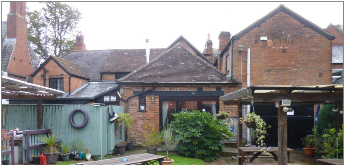
Figure 8: Rear elevation shows different phases of development including the garage to the right, gable projections, hipped extension with large glazed door, , lean-to, flat roofed extension to the left and outbuildings.
