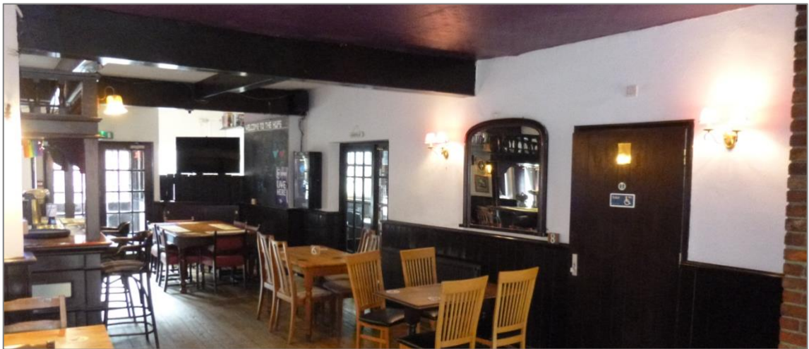
Figure 11: Area proposed to become residential, note large beams which are timber clad steel beams. Chimney breast to right will remain
