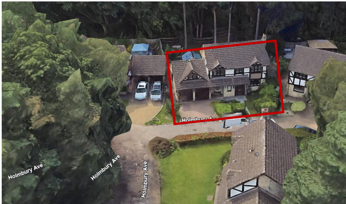
Partial hip to gable at neighboring property no. 24
