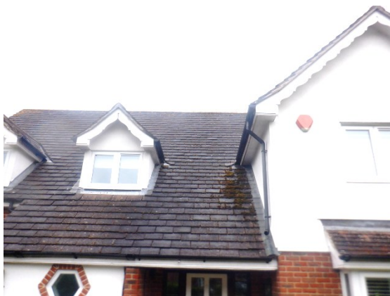
Photograph 5. Intact verge mortar across the gable and dormers (front elevation).
