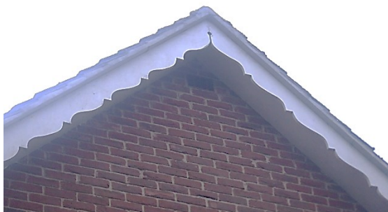
Photograph 12. Ornamental gap within the soffit at the apex of each gable (north elevation).
