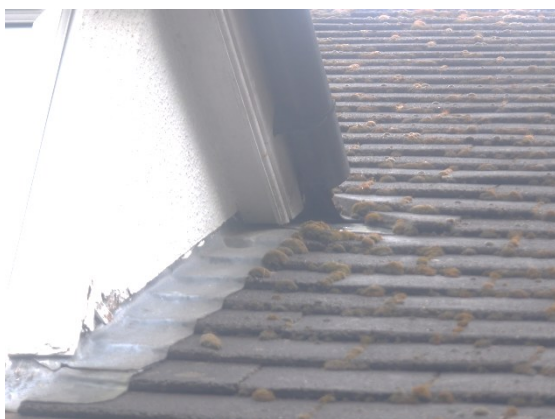
Photograph 10. Corners of front dormer windows sealed to the roof (front elevation).
