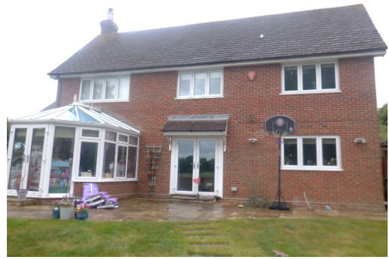
Photograph 2. Rear of property viewed from east.
