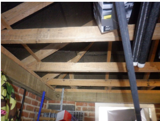
Photograph 23. Open roof garage with trussed beams and fully intact bitumen felt.
