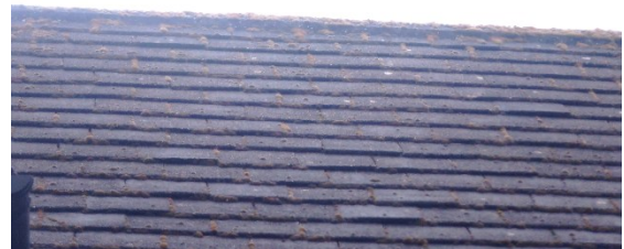
Photograph 4. Ridge mortar fully intact (rear elevation).
