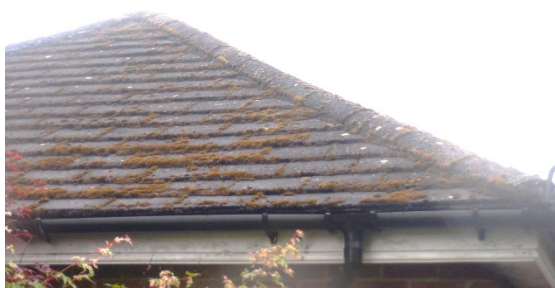
Photograph 14. Roof tiles and hip mortar fully intact and sealed across the garage.
