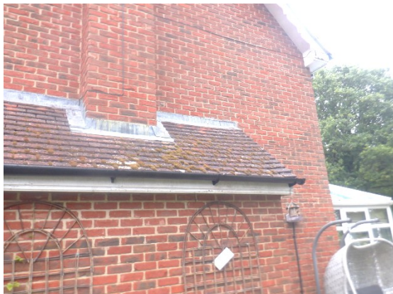
Photograph 6. Lead flashing sealed (south elevation).
