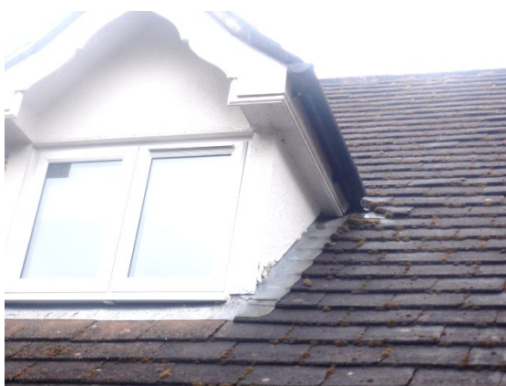
Photograph 8. Lead flashing sealed along dormer window (front elevation).
