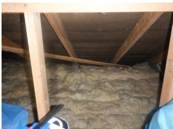
Photograph 19. Eaves mostly open with access to the timber soffit.
