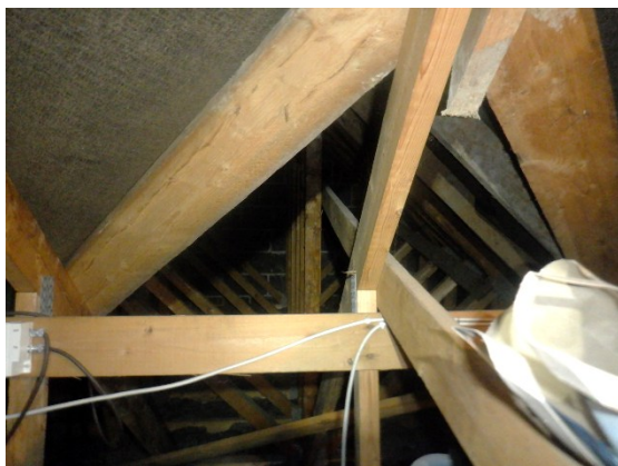
Photograph 16. Roof of trussed rafter construction.
