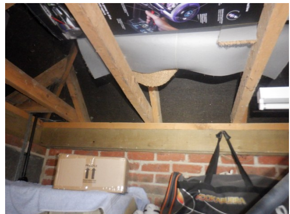
Photograph 24. Eaves sealed throughout the garage.
