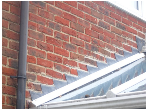
Photograph 7. Lead flashing sealed (rear elevation).
