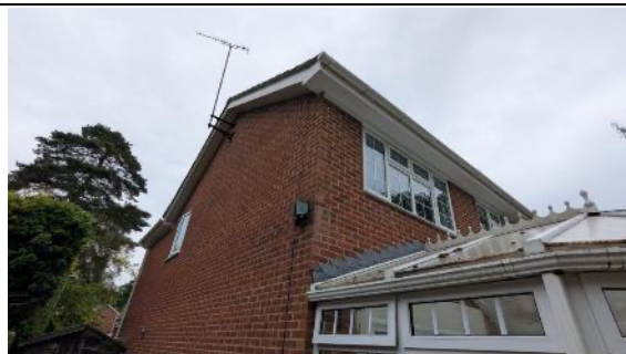
Photo 3: The southern gable end north and east elevation of the property. No potential bat roost features were found.
