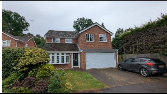
Photo 1: The front (south) elevation of the property. No potential bat roost features were found.
