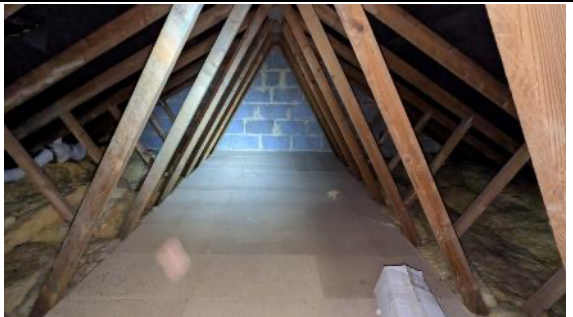
Photo 6: The east facing roof void.
