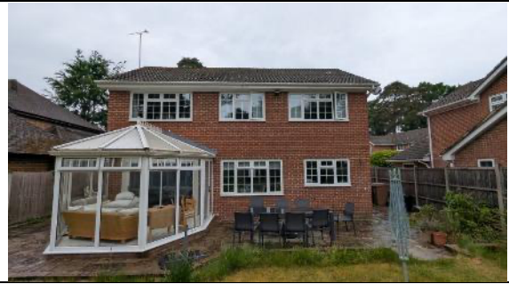
Photo 2: The north elevation of the property. No potential bat roost features were found.
