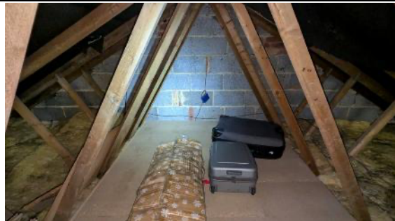
Photo 5: The west facing roof void of the attic was lined with insulated roof lining and had numerous cobwebs. No evidence of bats found.
