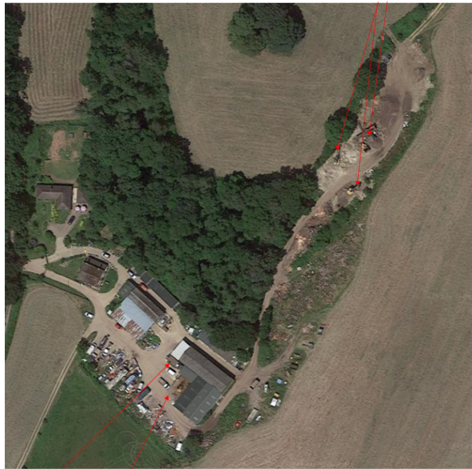
Operators cabin Vehicles in waste reception area
