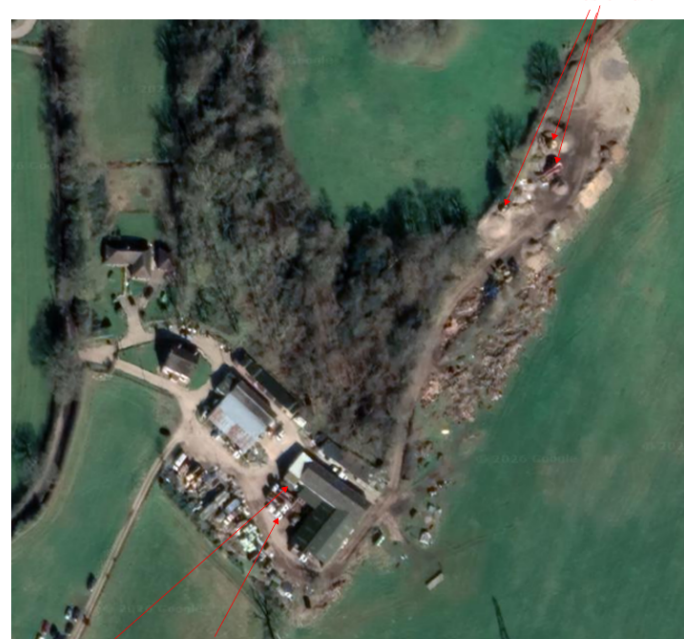
Operators cabin Vehicles reception area
