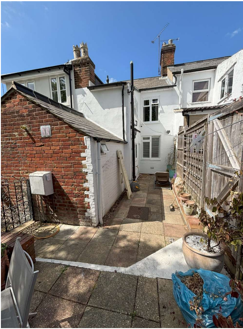
Photograph: 01 – Rear elevation of 42, Brook Street
