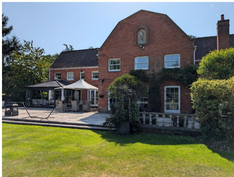
Existing Rear View from West with the dark grey solid roofed conservatory
