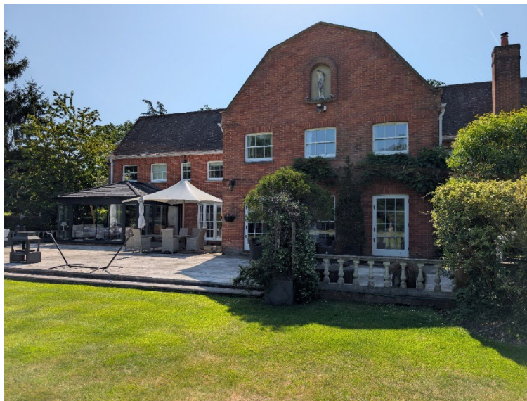
Existing Rear View from West with the dark grey solid roofed conservatory
