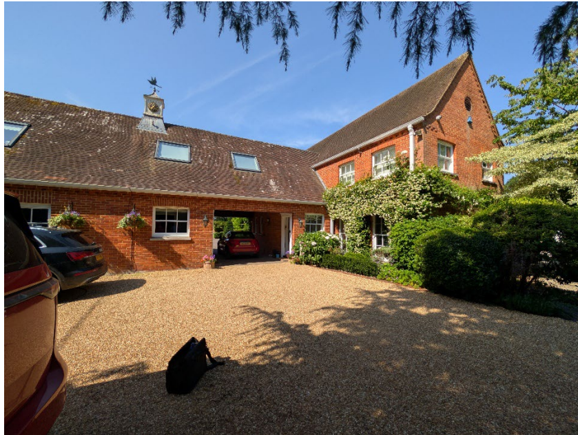
Clay Court viewed from the private drive to the east
