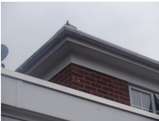
Photograph 7. Intact soffits tight to the brick of the property (north east elevation).
