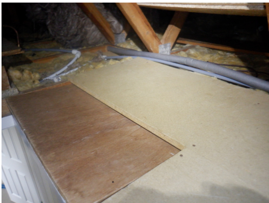
Photograph 16. Centrally boarded roof void.
