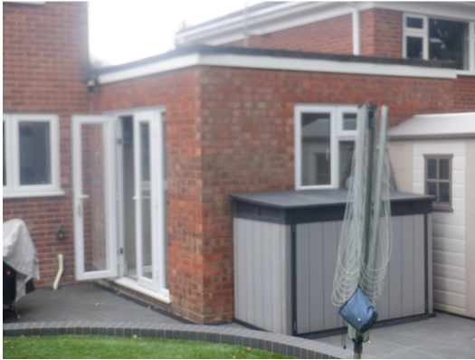
Photograph 9. Extension with bitumen roofing felt and uPVC bargeboards mostly tight.
