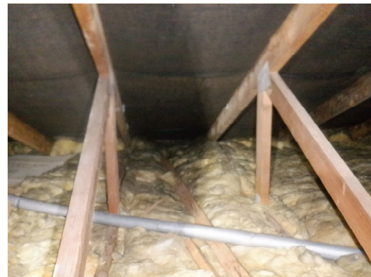
Photograph 17. Fibreglass filling the eaves of the roof void.
