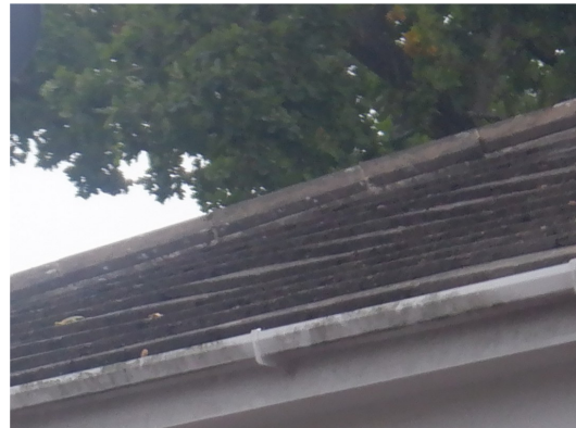
Photograph 4. Intact mortar between hip tiles and plain roof tiles (western elevation).
