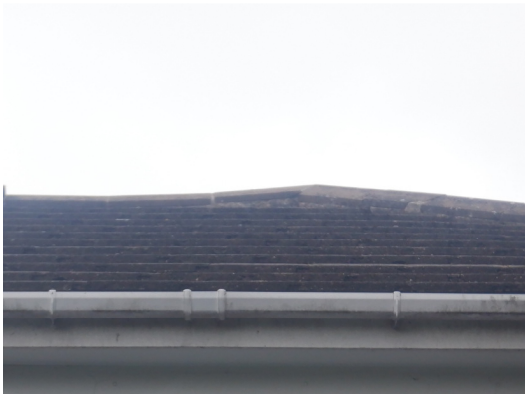
Photograph 3. Intact/tight plain roof tiles (eastern elevation).
