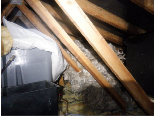
Photograph 18. Covered water tank (roof void).
