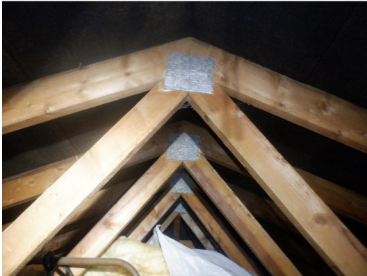
Photograph 14. internal view of the roof void..
