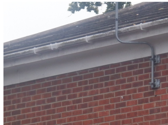
Photograph 8. Tight and intact barge boards around property (northern elevation).
