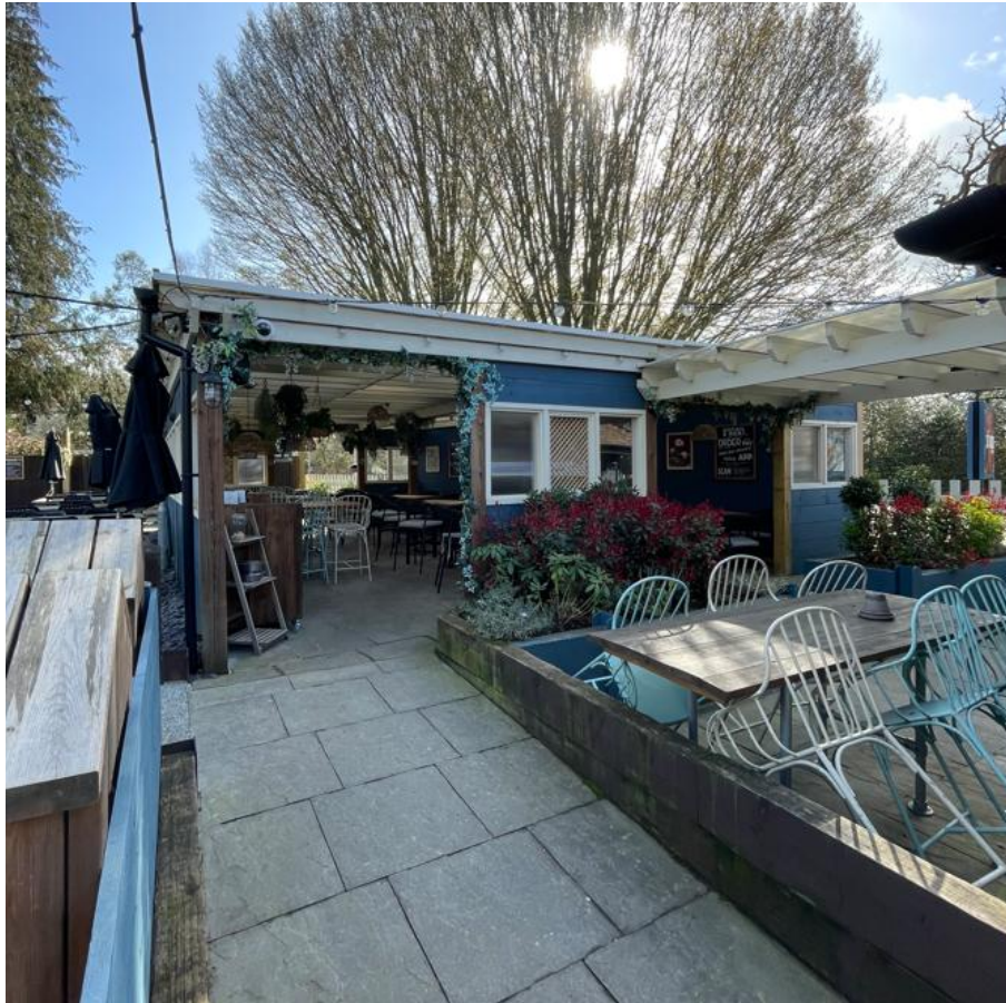
West elevation of enclosed customer seating area and covered walkway
