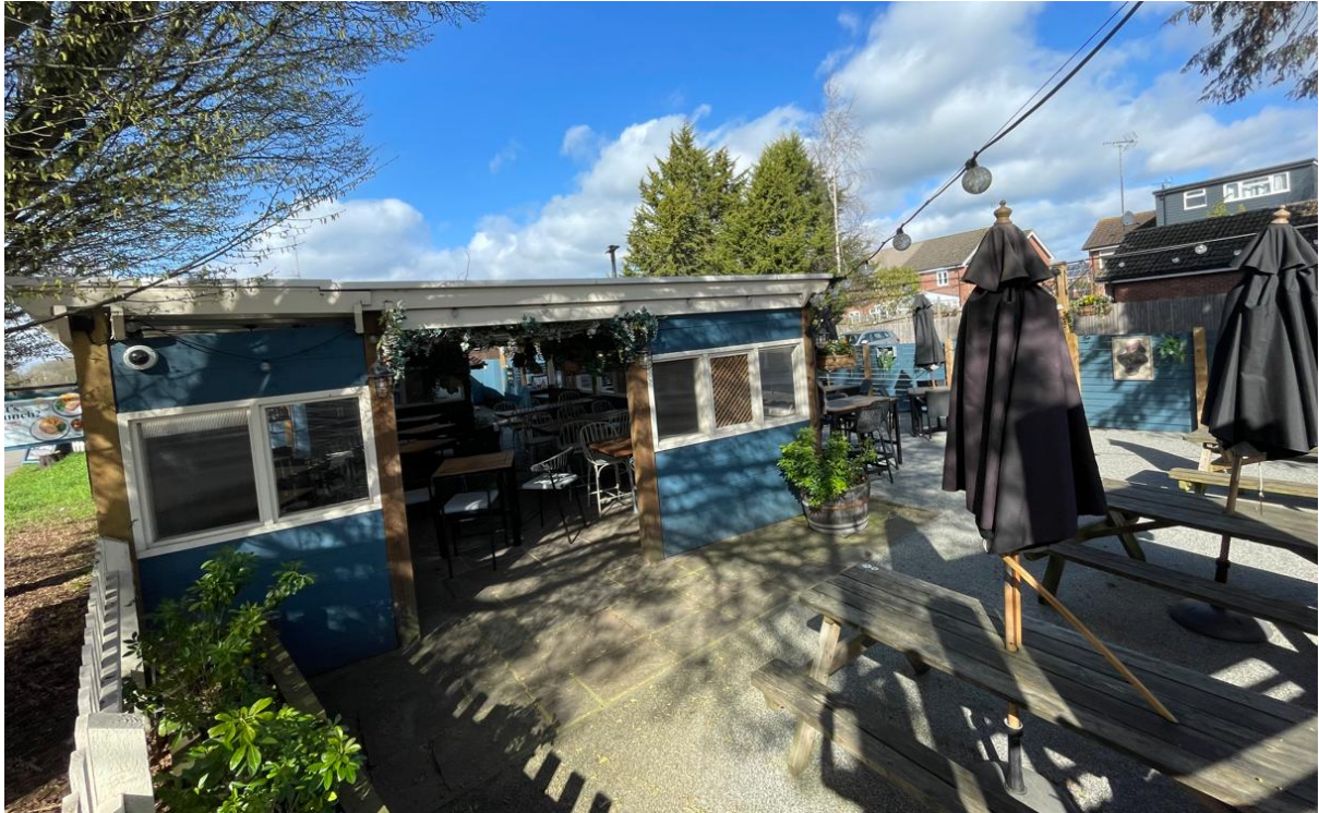
East elevation of enclosed customer seating area
