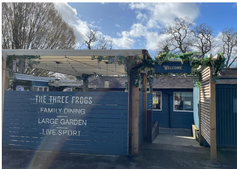
North elevation of pergola (with timber arbour to right side)
