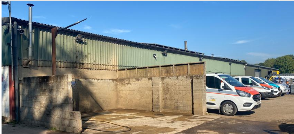
Eastern building (east façade). A new building will be constructed opposite.
