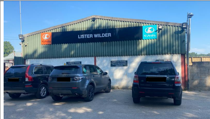
The Eastern building fronts onto White House Lane (south façade). Three budget luminaire floodlights, tilted.
