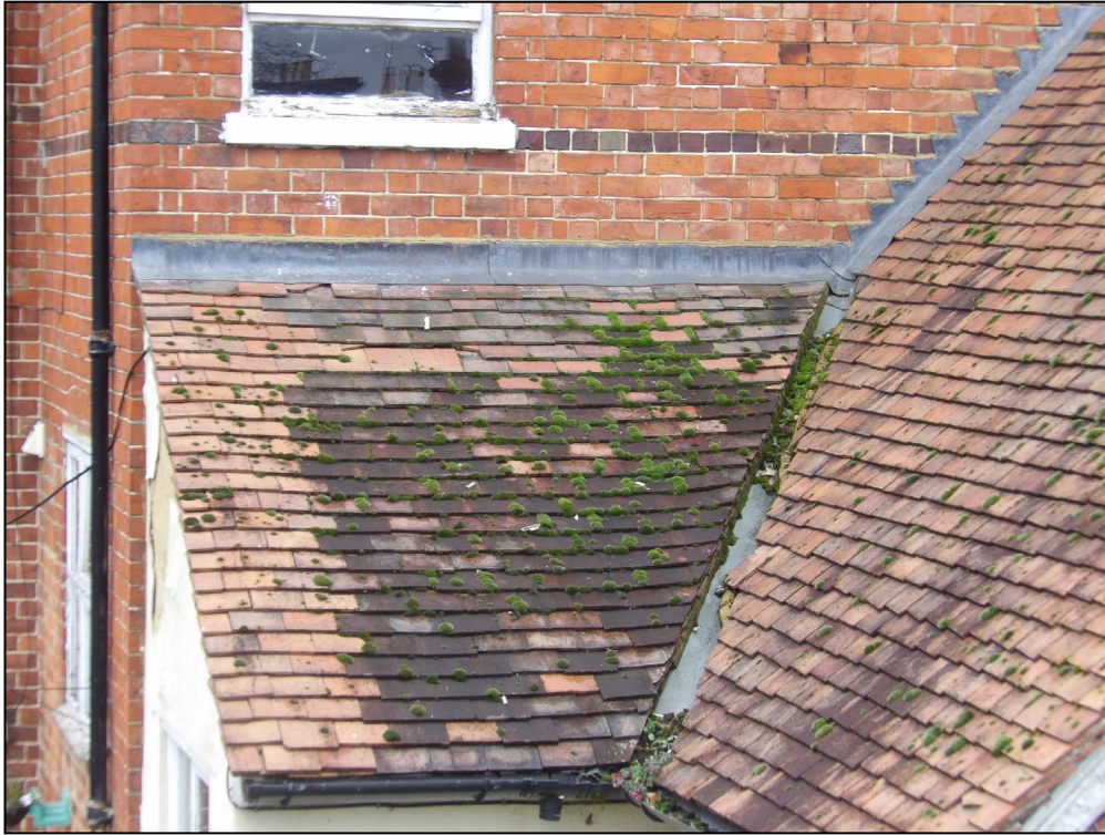
Figure 11. Broken roof tiles rear extension. Arlington, Basingstoke Road, Spencers Wood. 10.12.24
