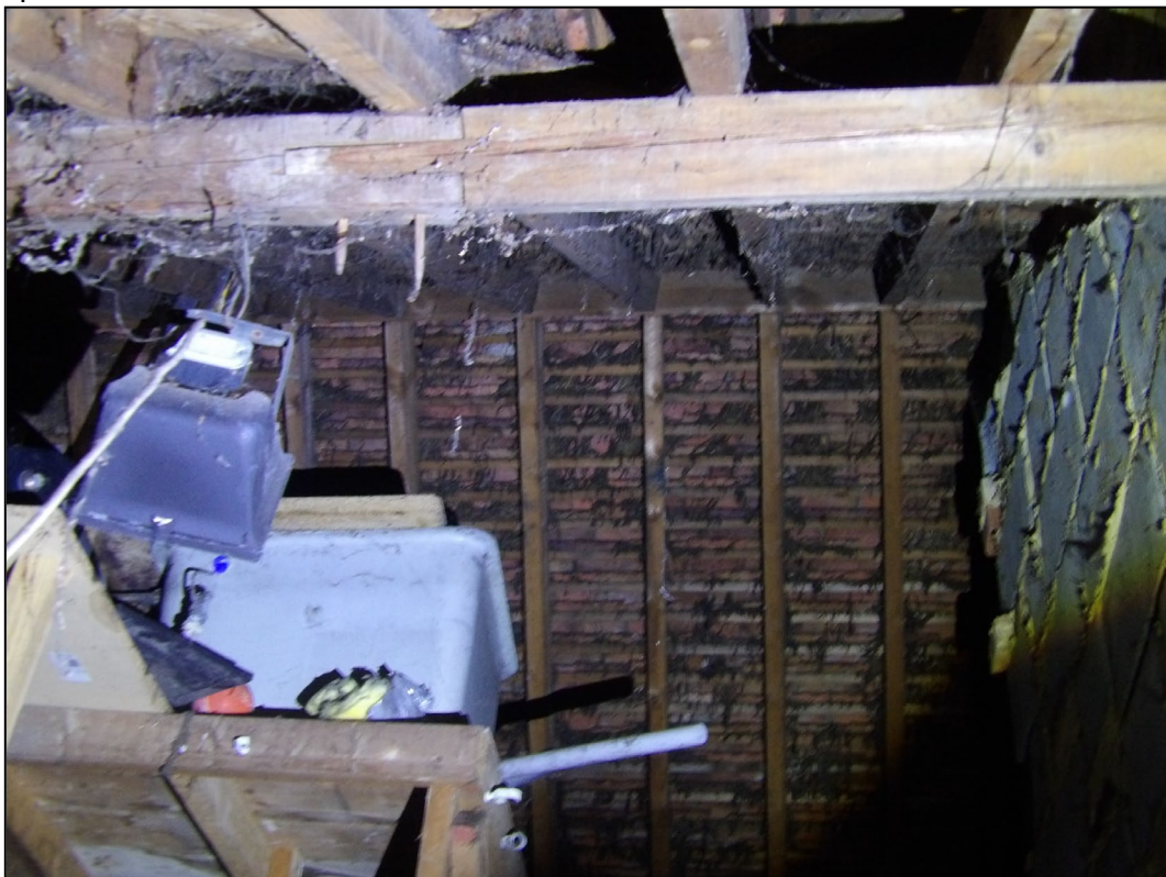
Figure 15. Example of loft space and unlined roof tiles. Arlington, Basingstoke Road, Spencers Wood. 10.12.24
