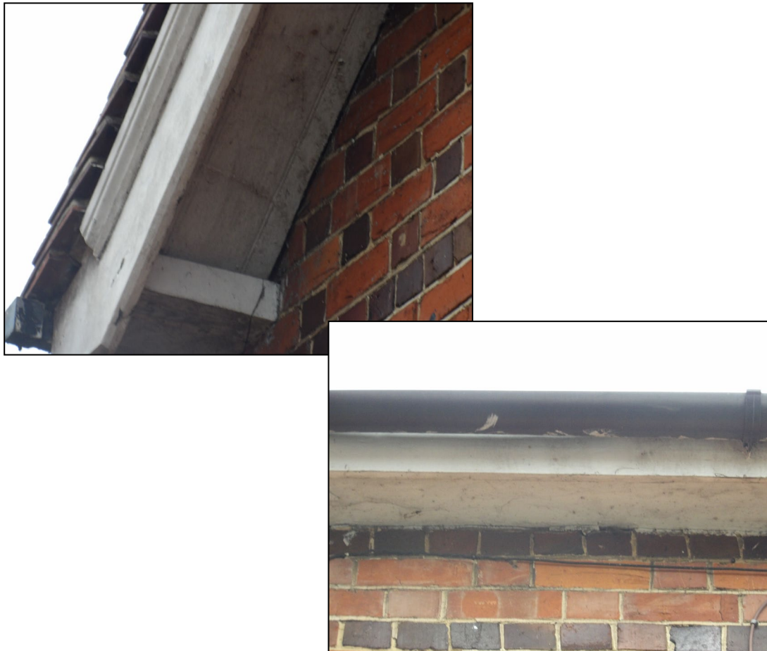
Figure 8. Example sealed soffits/fascias. Arlington, Basingstoke Road, Spencers Wood. 10.12.24
